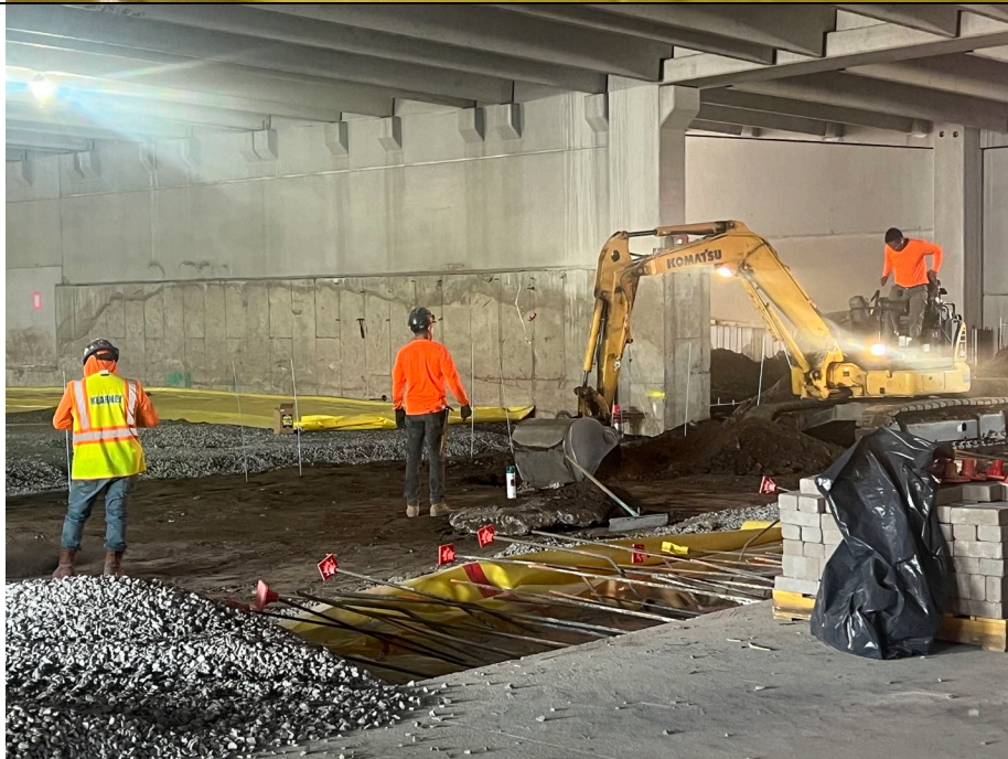
Photo 4: Looking west, Kingdom excavating to unearth existing pile caps in grid B1.
