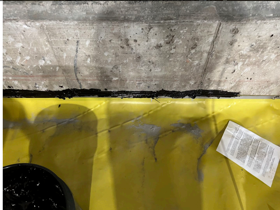
Photo 2: View of vapor barrier being sealed against existing concrete wall in accordance with manufacturer's specifications.
