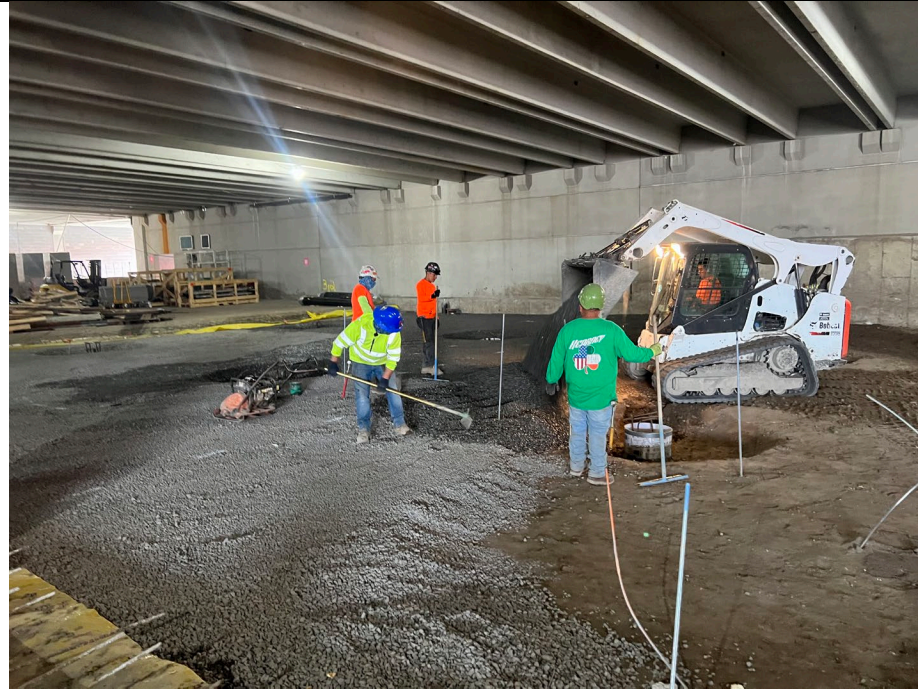
Photo 1: Looking southwest, Kingdom continues backfilling with \frac{3}{4} " stone from Tilcon in grids B2 and B1.
