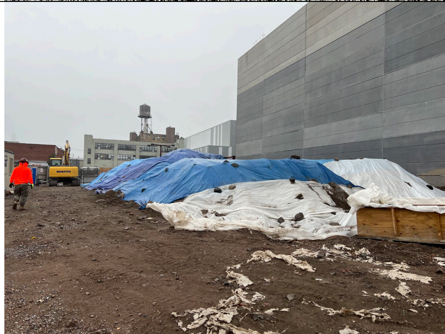
Photo 4: View of cover over temporary stockpile.
