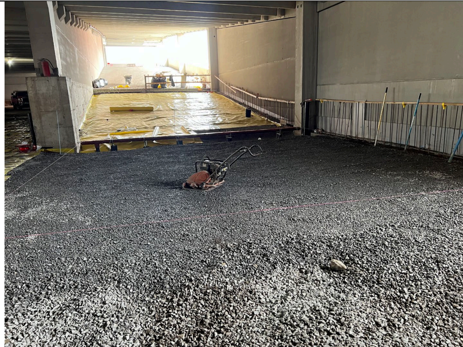
Photo 3: Looking south, view of vapor barrier installation and backfill in grid B1.
