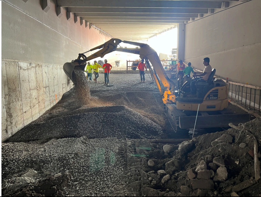
Photo 1: Looking south, Kingdom backfilling with ¾" stone from Tilcon in grid B1.
