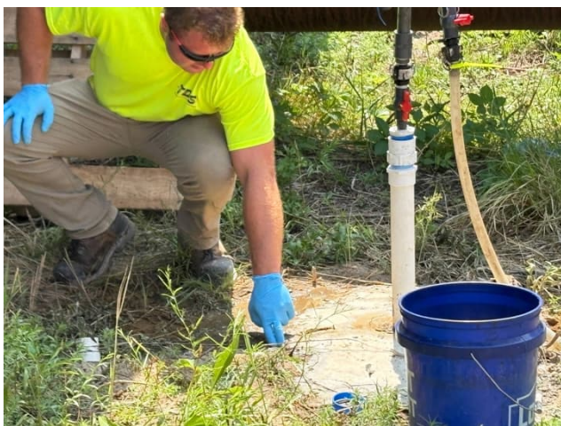
Photo 3 – Treatment surfacing/ daylighting at IW-12.
