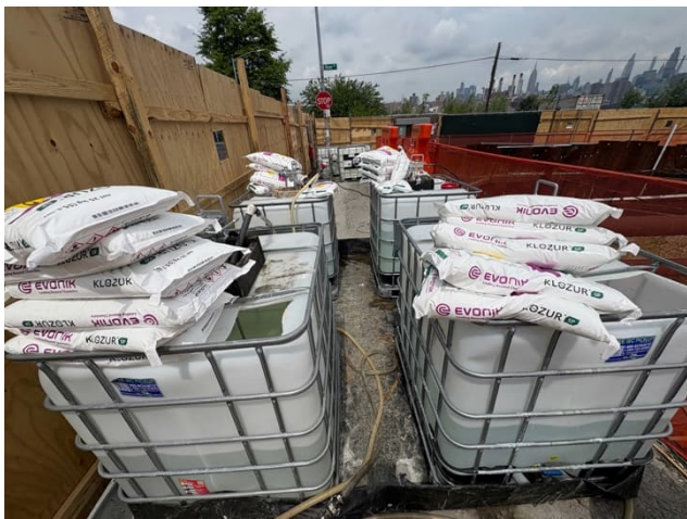
Photo 1 – ISCO treatment mixing and injection water totes.
