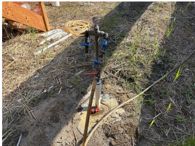
Photo 2 – ISCO treatment pumping at IW-9
