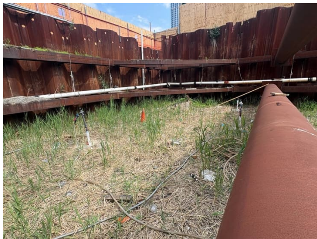
Photo 2 – Chemical injections at IW-3 and IW-5
