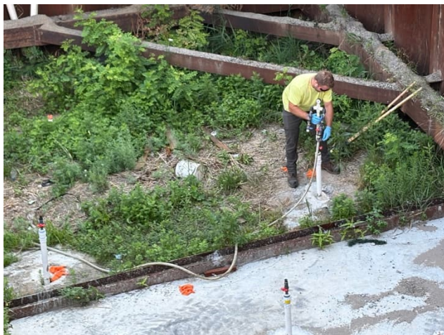
Photo 1 – Hook up of injection well head to IW- 14.
