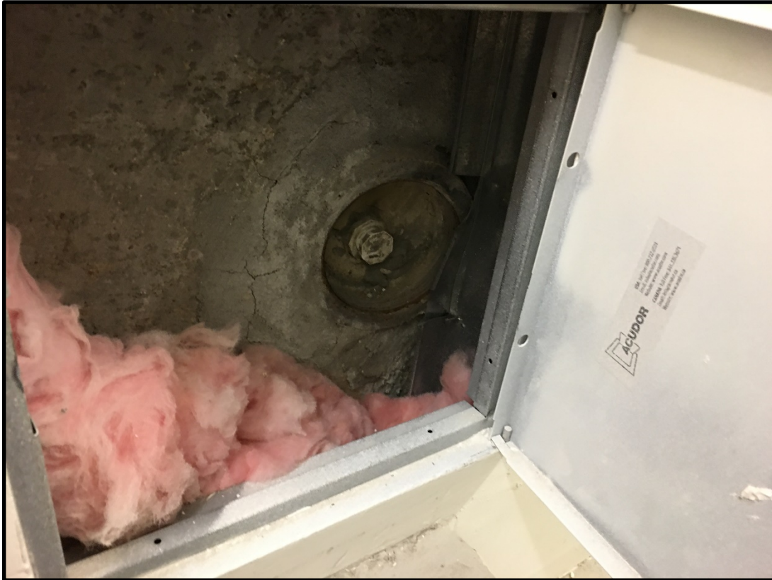
Photograph 7: Photo of MP-1 (west SSDS) within lock box within private stairwell leading from first floor to the cellar.
