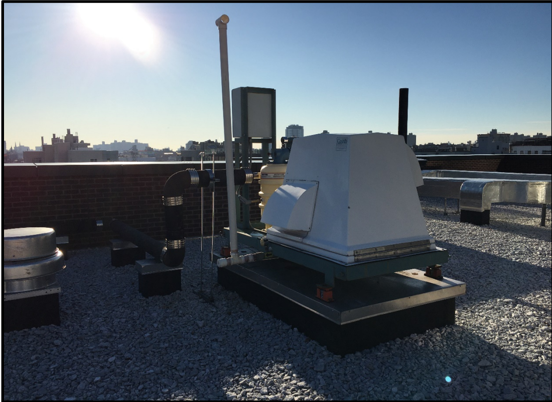
Photograph 10: SSDS Blower 1 and associated run of piping (left).
