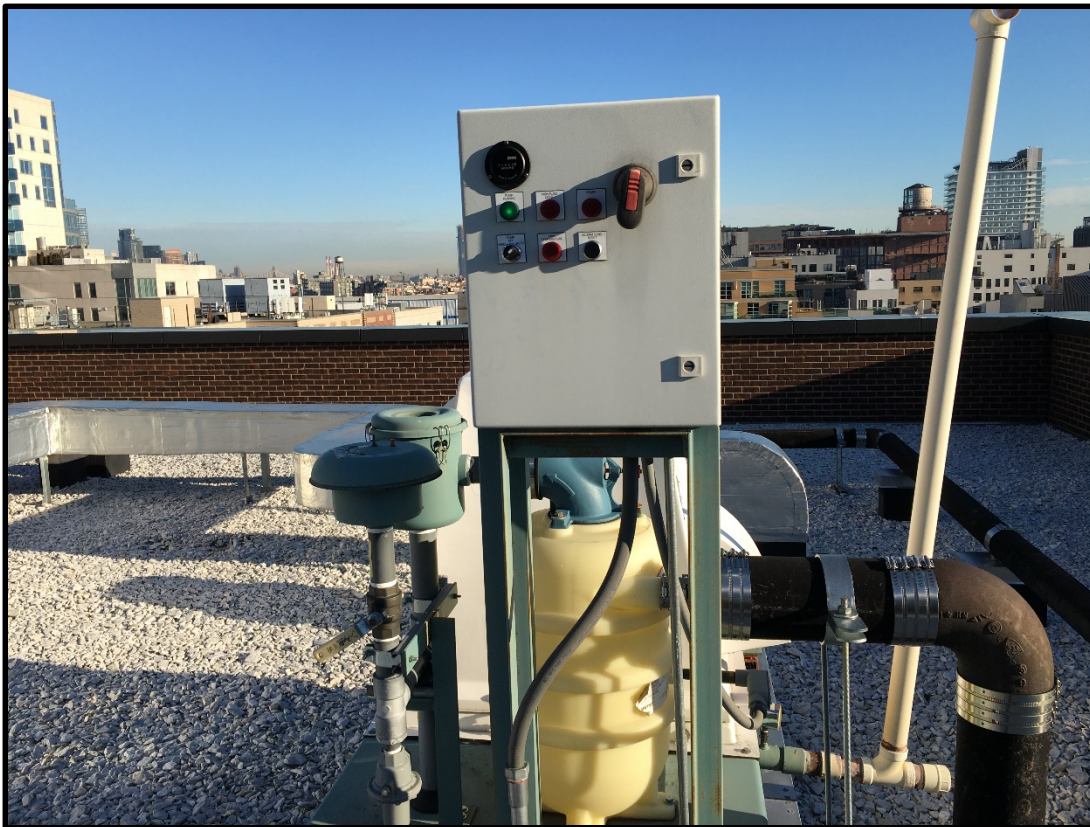
Photograph 12: Photo of SSDS Blower 2 (east) control panel upon arrival.
