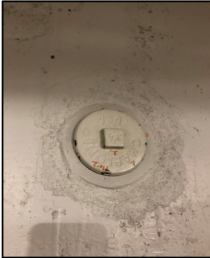
Photograph 11: View of MP-2 (east SSDS) after field pressure test.
