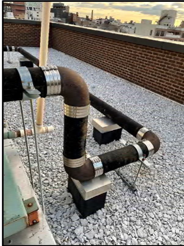
Photograph 10: Representative view of aboveground piping located on the roof leading to the SSDS Blower 1. All piping and couplings were intact.
