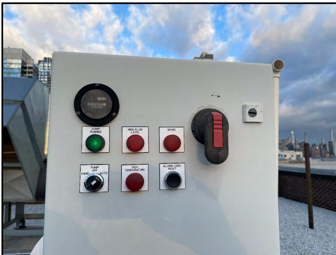
Photograph 12: Photo of SSDS Blower 2 (east) control panel.
