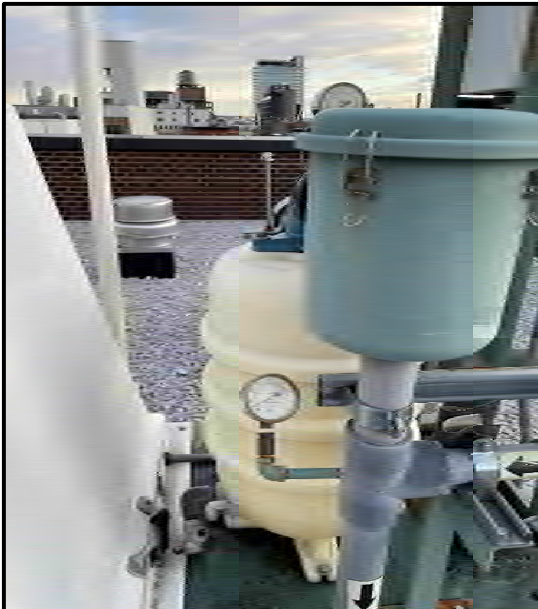
Photograph 14: Photo of SSDS Blower 2 (east) inlet and knockout tank vacuum readings.
