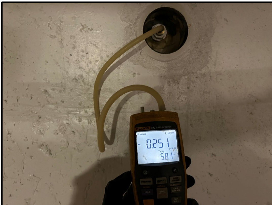
Photograph 6: View of MP-2 (east SSDS) field pressure test.
