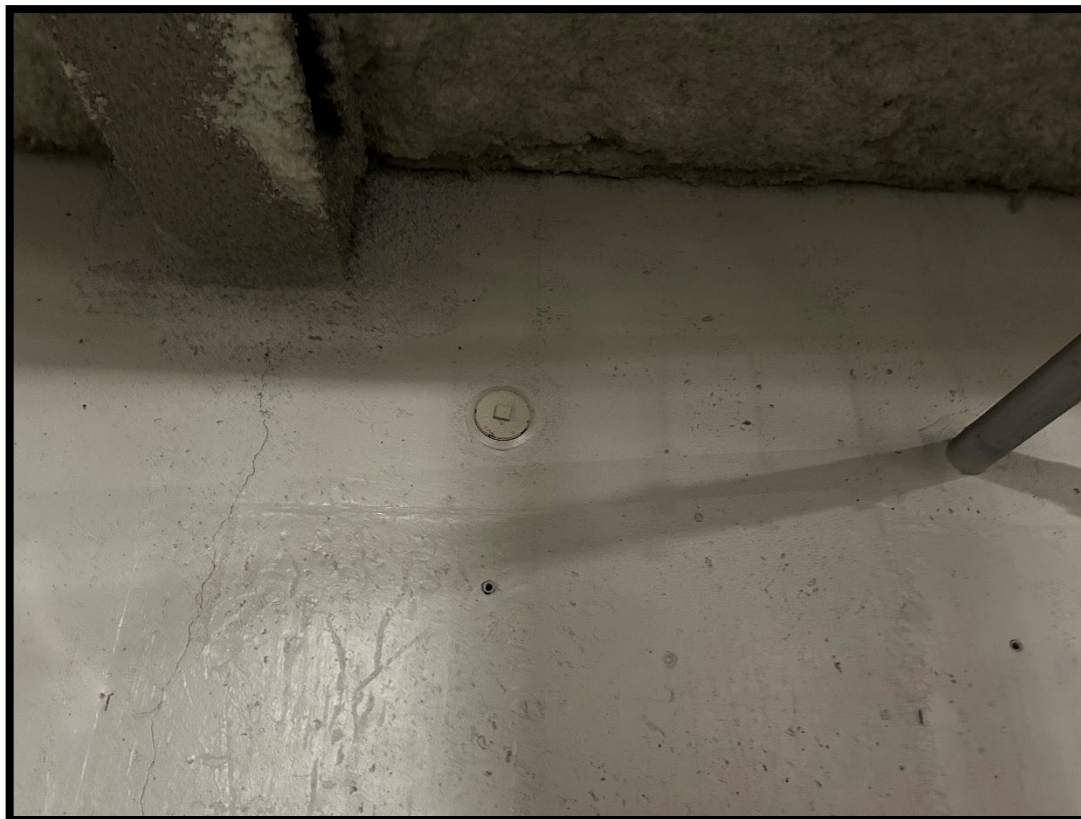
Photograph 4: View of MP-2 location and protective cover located in on the east side of the northern wall of the cellar parking garage.
