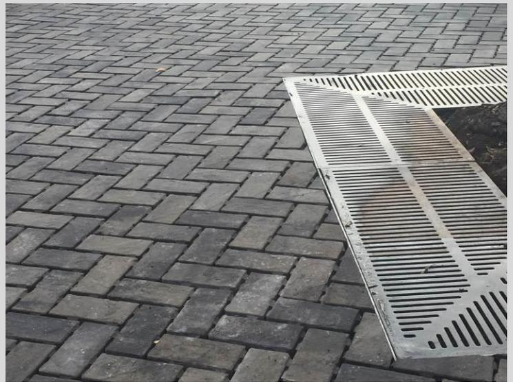
PHOTO 10: Details of the porous pavers and final work.
