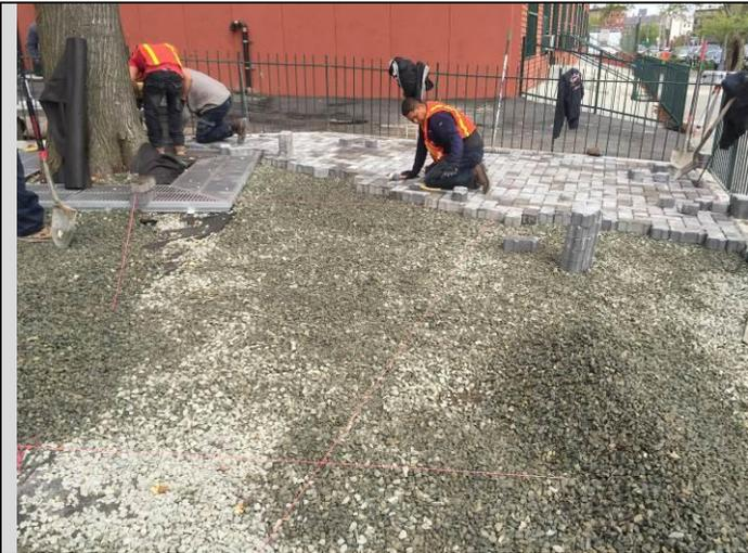
PHOTO 7: Another view of the porous pavers and tree grate.
