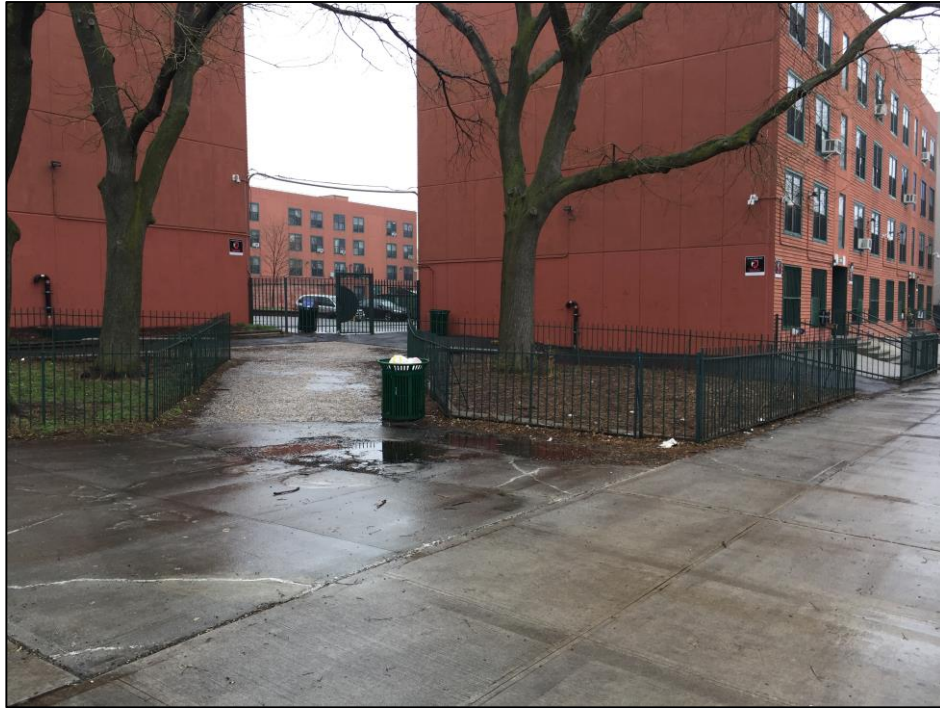
Photo 1: Looking northeast towards BCP Site No. C224162
