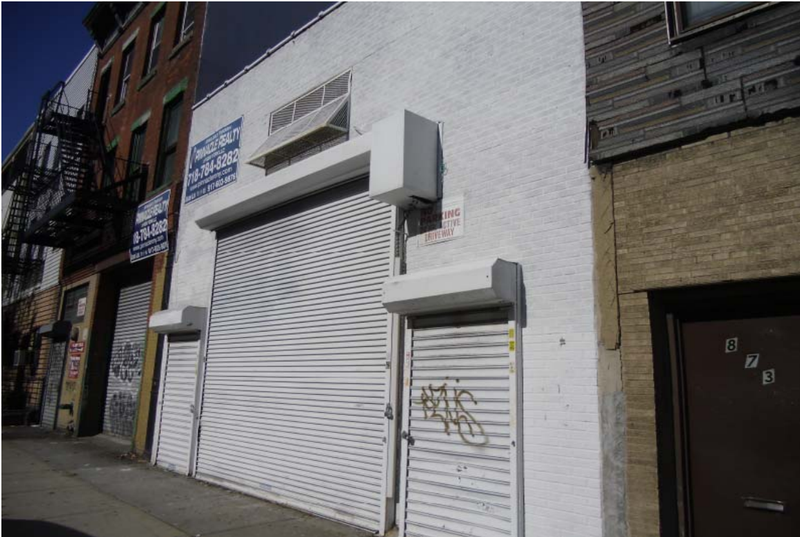
Photo 6 – From left to right: View of 869 Grand Street, 871 Grand Street (subject site), and 873 Grand Street.
