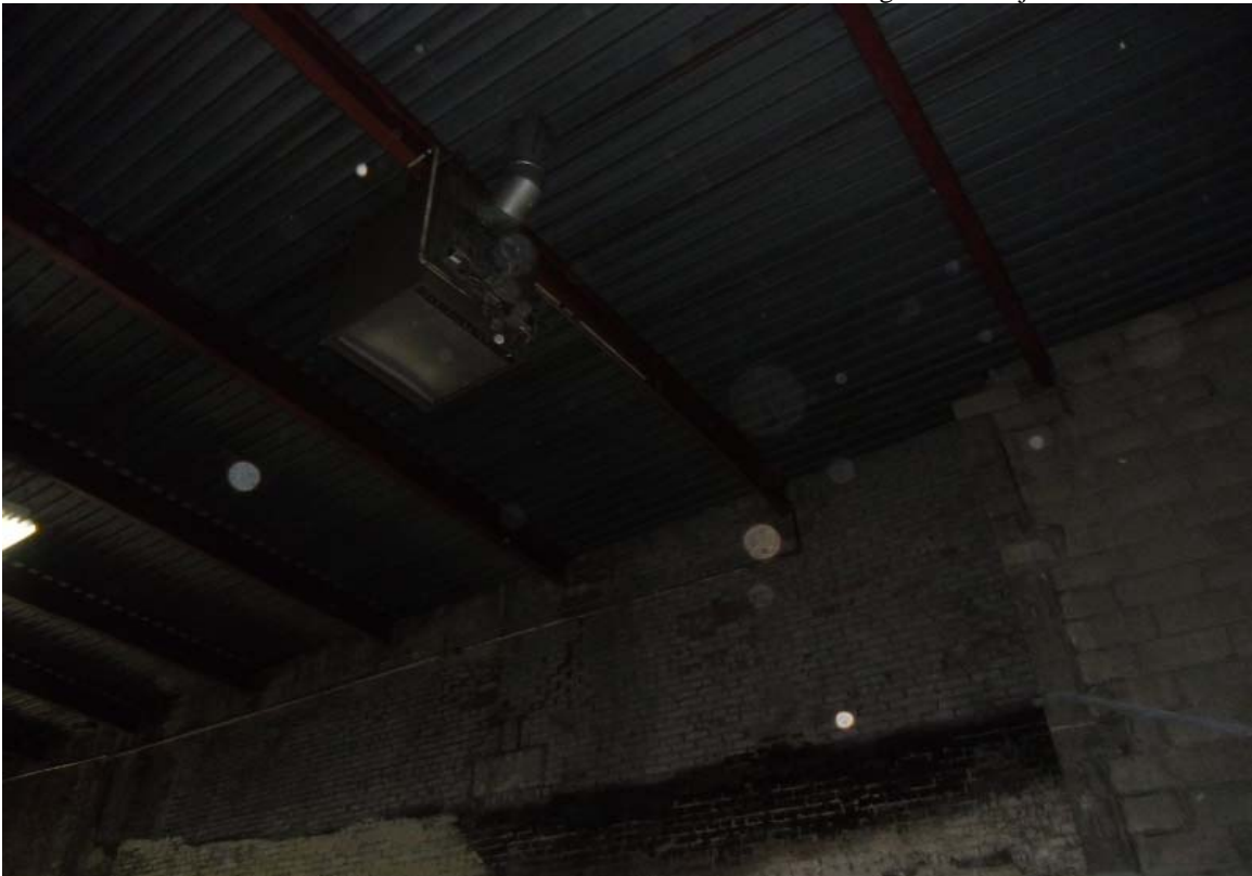
Photo 5 – View of gas powered space heater hanging in building on subject site.
