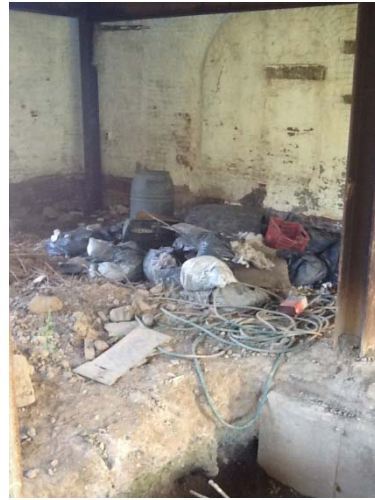
View of concrete foundations of the unfinished construction
