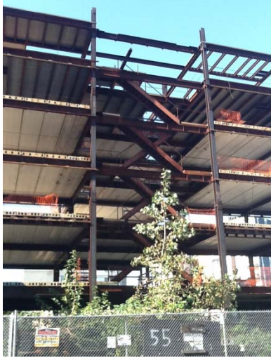
View of the 6-story steel frame construction
