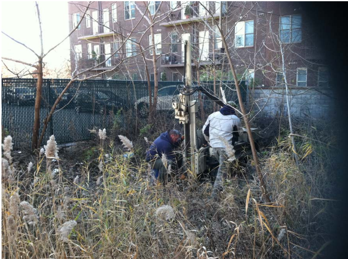
Fig 4. View of boring B-4 advanced on the subject property.
