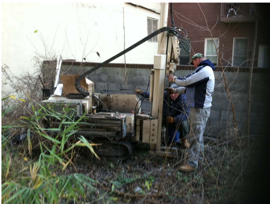
Fig 6. View of boring B-6 advanced on the subject property.
