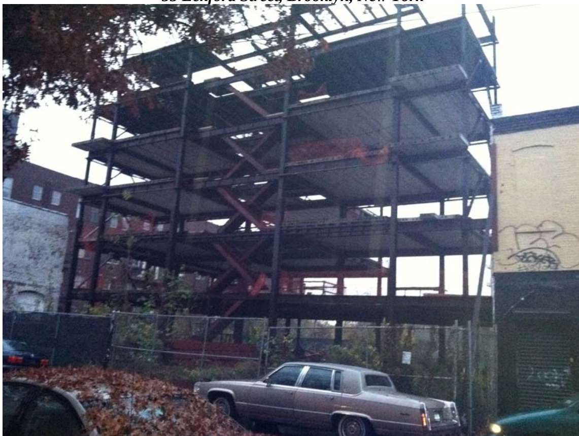
Fig 1. View of Subject Property located at 55 Eckford Street, Brooklyn, NY.
