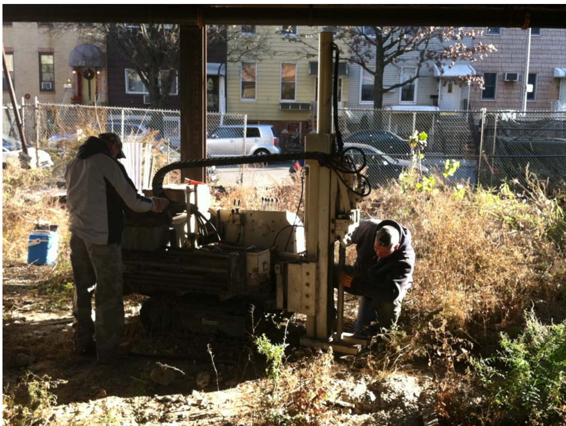
Fig 2. View of boring B-1 advanced on the subject property.
