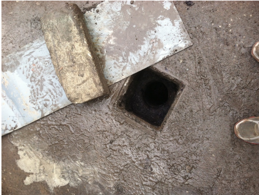
Photo 15: View of FD015 cleaned out.
