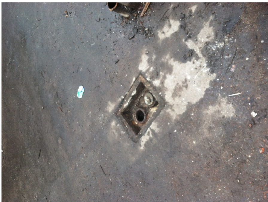
Photo 12: View of FD011 cleaned out.
