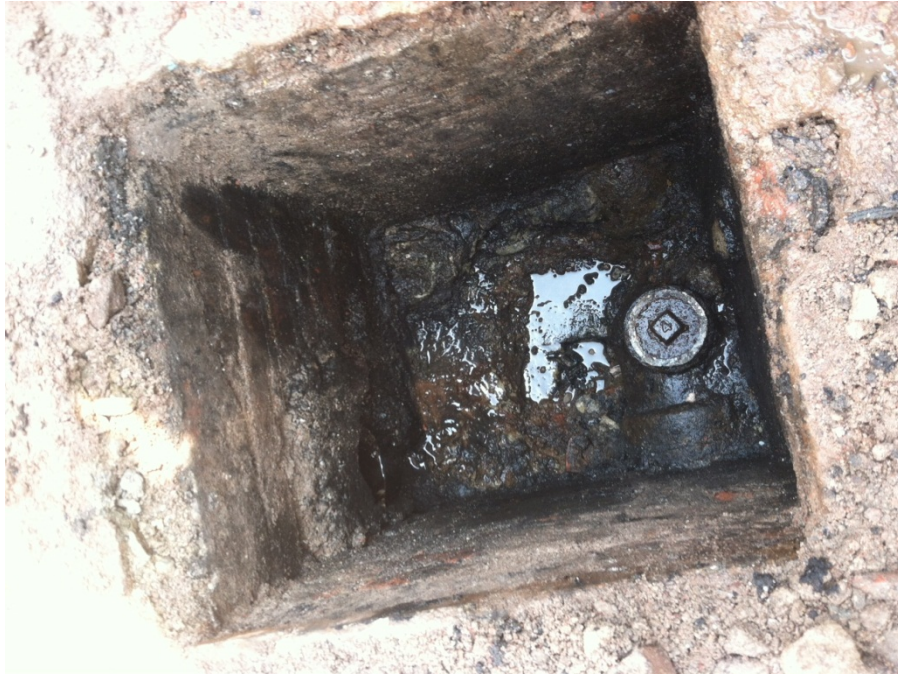
Photo 5: View of FD004 cleaned out.
