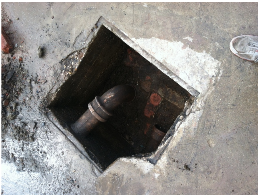
Photo 6: View of FD005 cleaned out. Note the earthen bottom.
