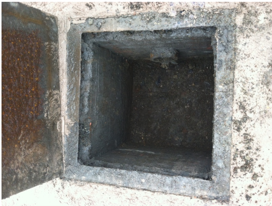
Photo 10: View of FD009 cleaned out.
