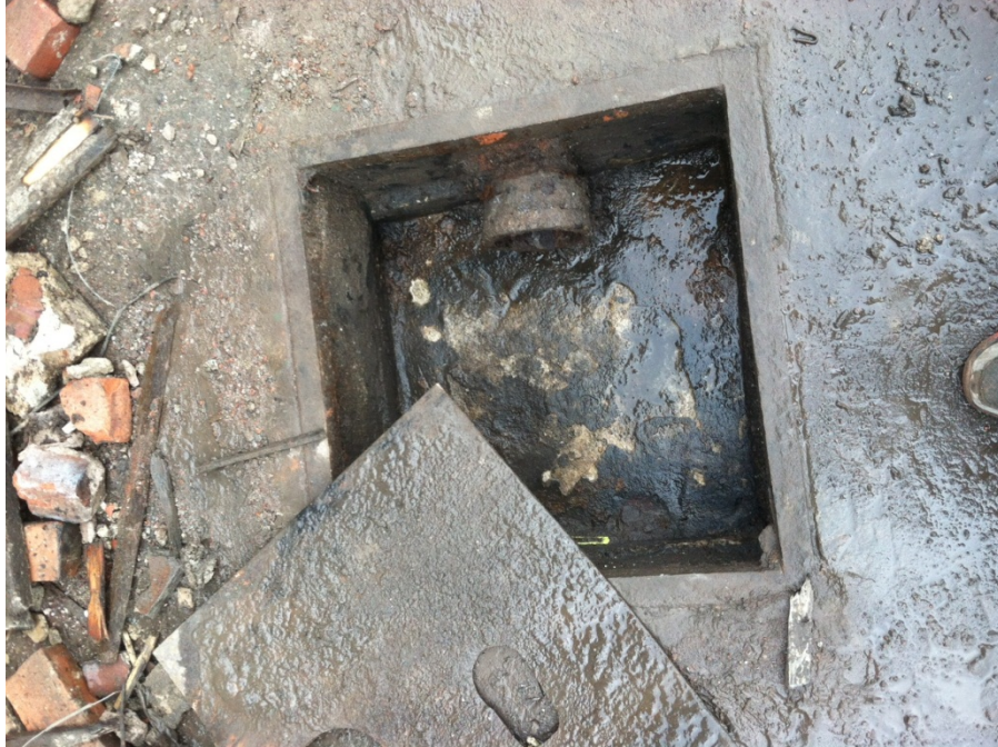
Photo 3: View of FD002 cleaned out.
