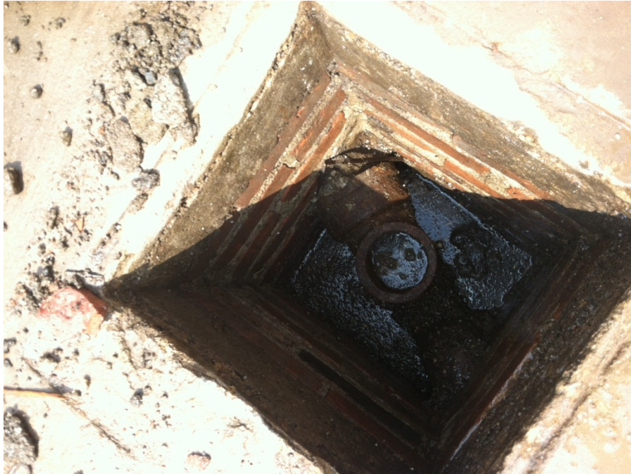
Photo 7: View of FD006 cleaned out.
