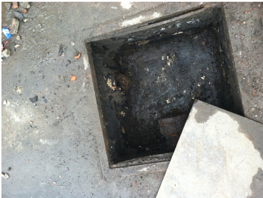
Photo 4: View of FD003 cleaned out.
