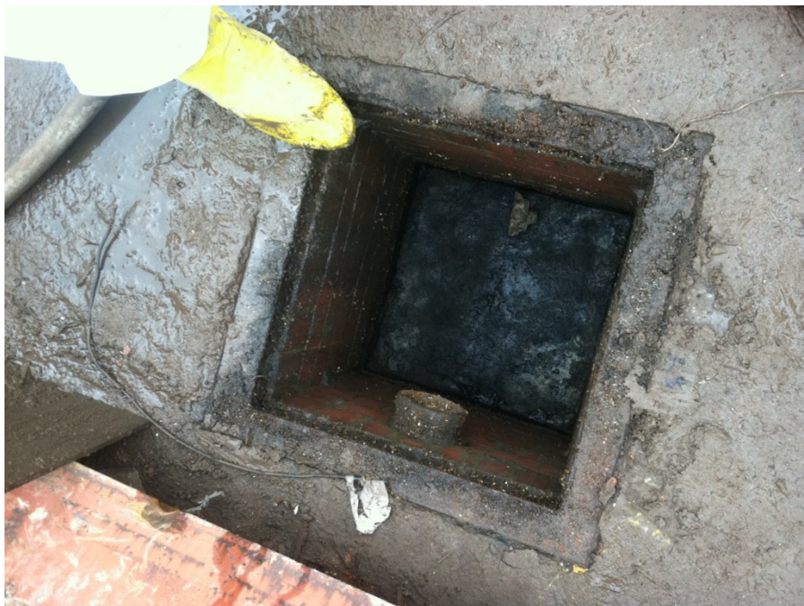
Photo 8: View of FD007 cleaned out.
