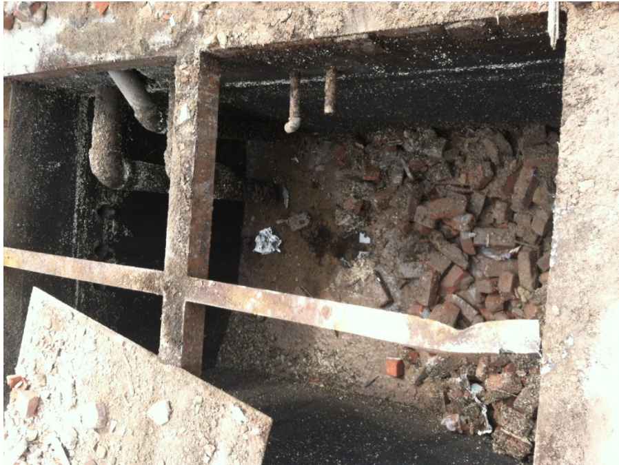
Photo 1: View of concrete vault with liquid removed and sediment removed.
