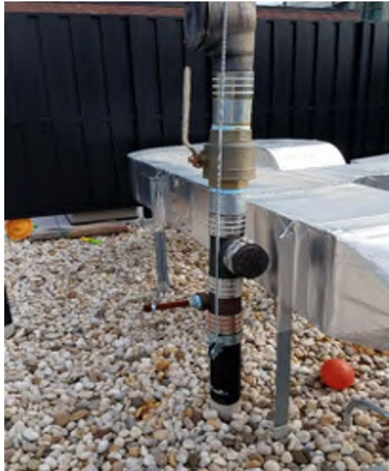
Photo 11: V3 riser and sample port in good condition, facing east. 27 February 2019.
