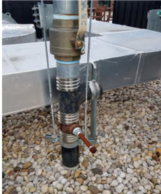
Photo 5: V1 riser and sample port in good condition, facing east. 27 February 2019.
