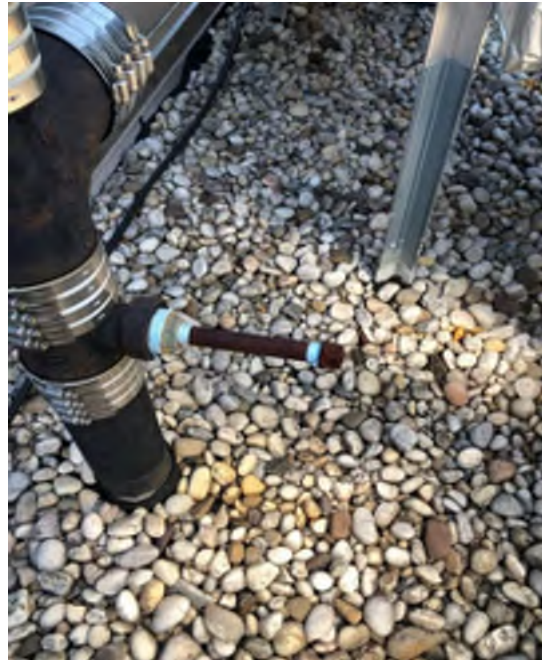
Photo 10: V4 riser and sample port in good condition, facing east. 8 April 2021.
