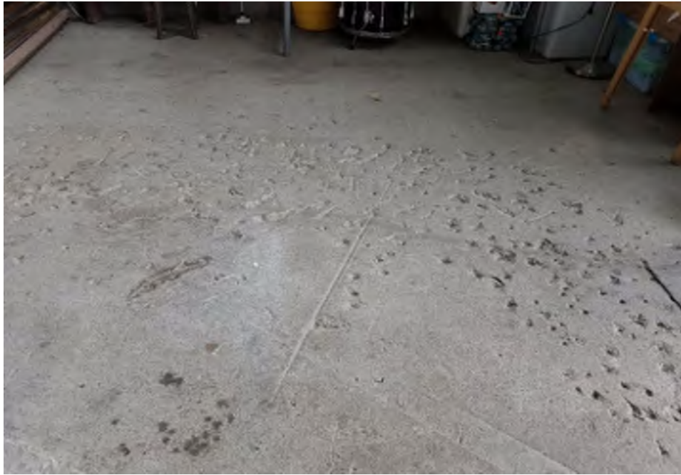
Photo 15: Hairline/surficial cracks observed within the boat house, facing southeast. Cracks did not breach to the subsurface. 27 February 2019.
