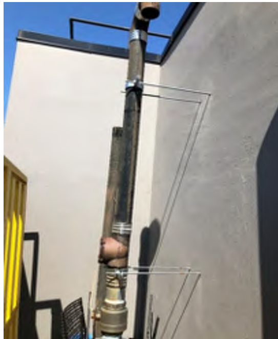
Photo 14: V6 riser and sample port in good condition, facing northwest. 8 April 2021.
