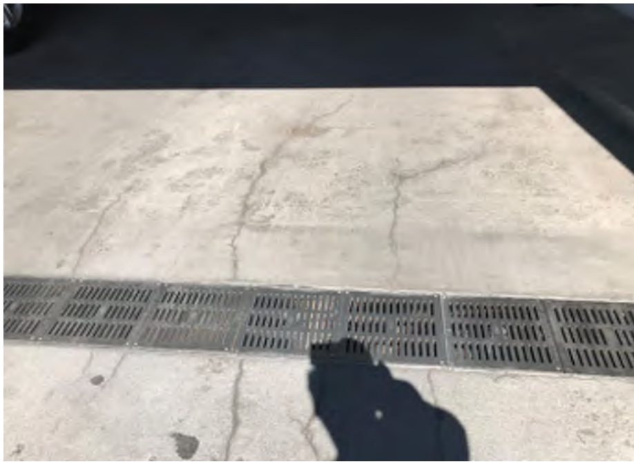
Photo 9: Typical hairline/surficial crack observed in the parking garage, facing north. Cracks did not breach to the subsurface. 30 March 2021.
