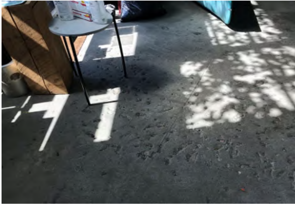
Photo 15: Hairline/surficial cracks observed within the boat house, facing southeast. Cracks did not breach to the subsurface. 30 March 2021.
