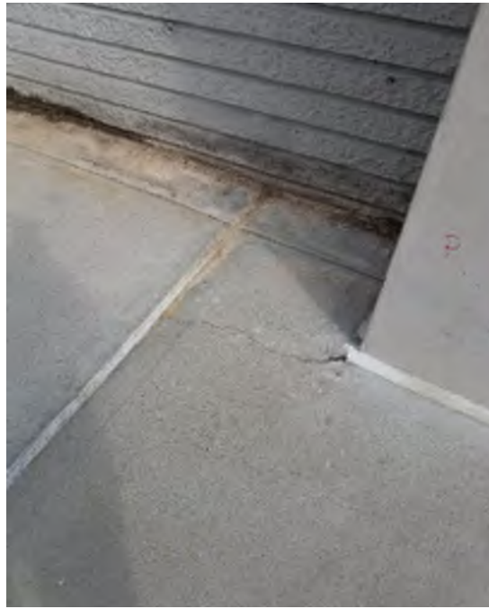
Photo 3: Typical hairline/surficial crack observed on sidewalks, facing northeast. Cracks did not breach to the subsurface. 27 February 2019.
