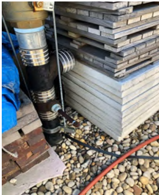
Photo 12: V5 riser and sample port in good condition, facing southeast. 8 April 2021.
