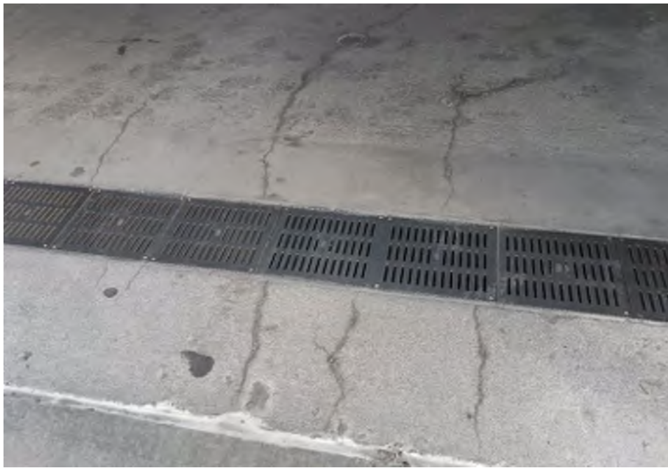
Photo 9: Typical hairline/surficial crack observed in the parking garage, facing north. Cracks did not breach to the subsurface. 27 February 2019.
