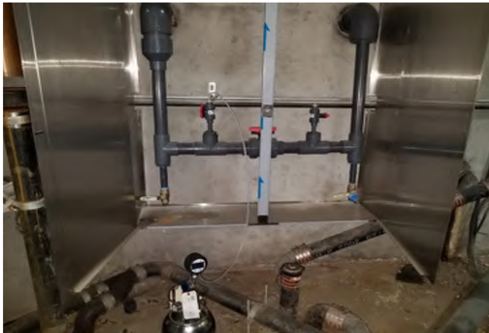
Photo 8: V2 subgrade sampling port in good condition, facing north. 27 February 2019.
