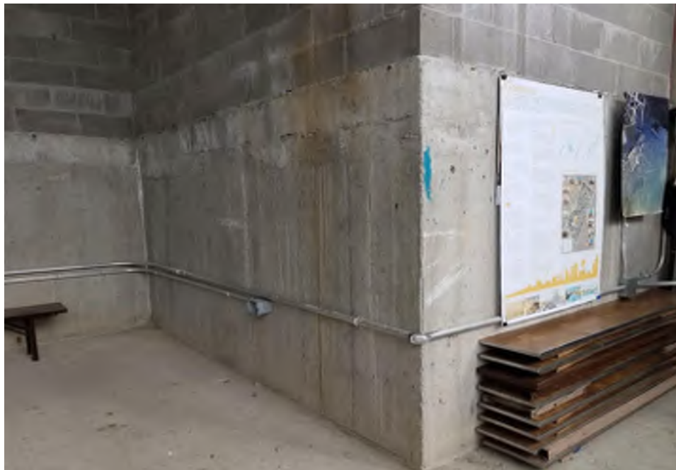
Photo 16: Concrete foundation wall (beneath first floor slab) in subgrade boathouse located within the southern portion of the building, facing east. 27 February 2019.
