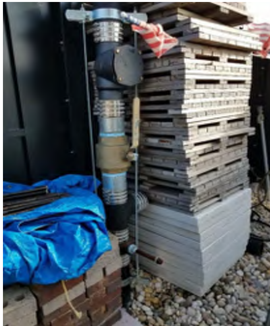
Photo 17: V5 riser and sample port in good condition, facing southeast. 27 February 2019.
