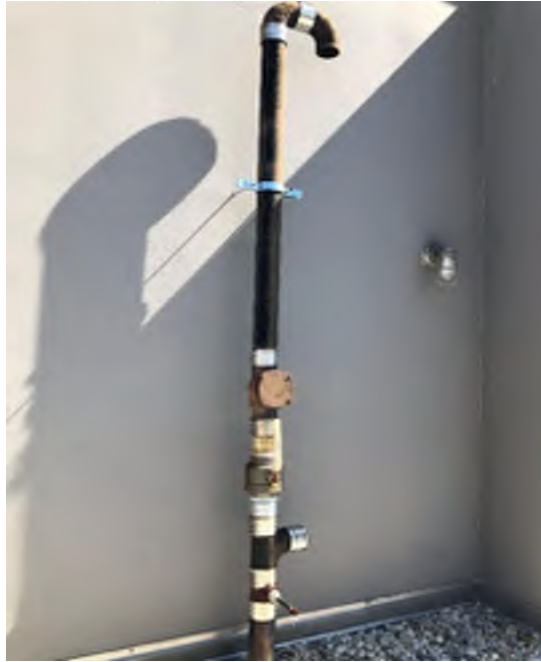
Photo 3: V2 riser in good condition, facing northeast. 8 April 2021.
