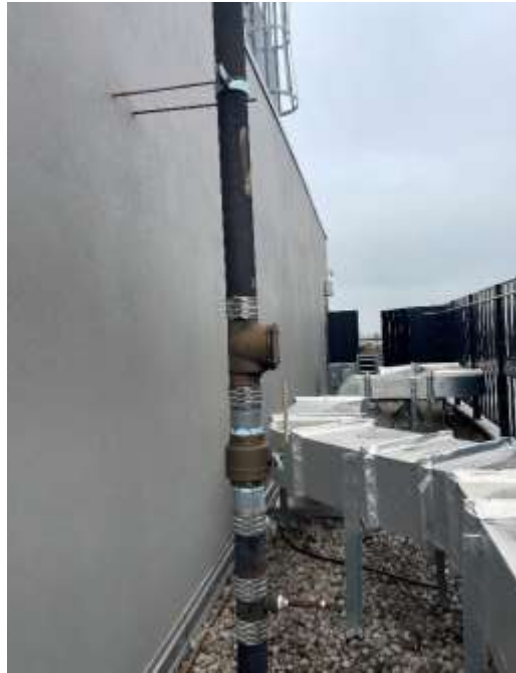
Photo 7: V4 riser in good condition, facing west. 02 March 2023.
