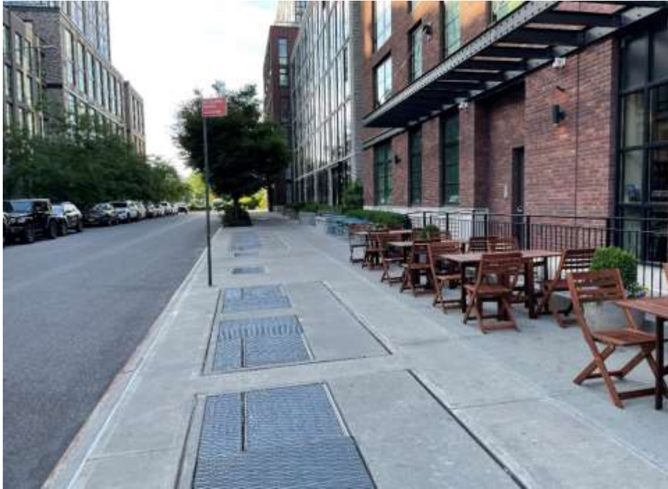
Photo 1: 1st Street sidewalk, facing southeast. 20 June 2022.
