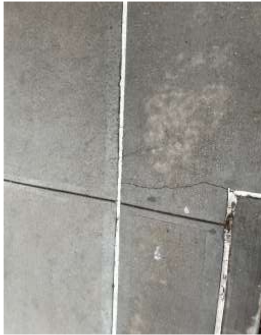
Photo 9: Typical hairline/surficial crack observed, facing north. Cracks did not breach to the subsurface. 02 March 2023.
