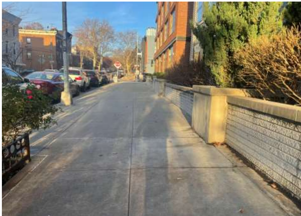
Photo 2: 2nd Street sidewalk, facing northwest. 05 December 2023.
