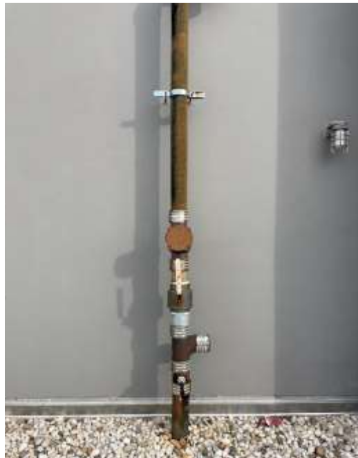
Photo 7: V4 riser in good condition, facing west. 05 December 2023.
