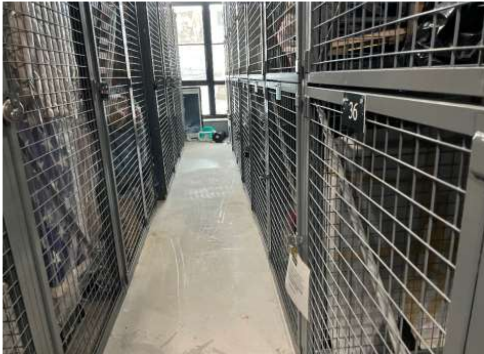
Photo 16: First floor concrete slab in tenant storage space, facing southwest. 02 March 2023.
