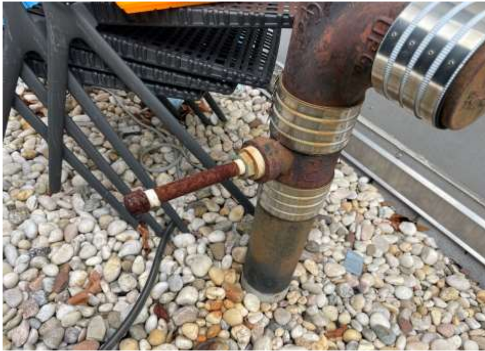
Photo 13: V6 riser and sample port in good condition, facing northwest. 05 December 2023.
