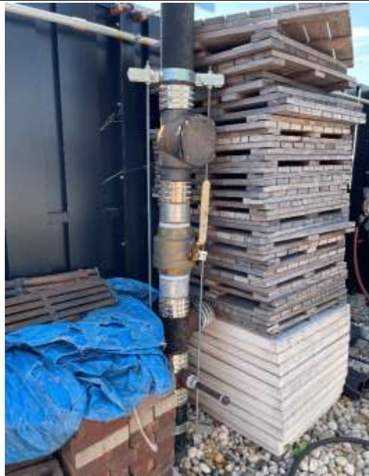
Photo 9: V5 riser in good condition, facing southeast. 20 June 2022.
