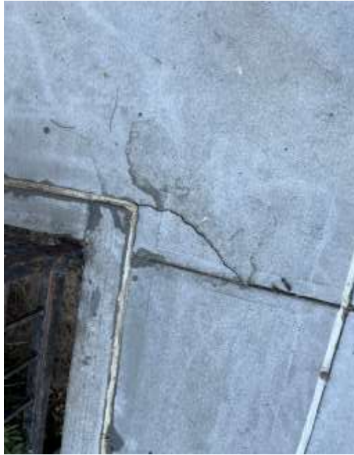
Photo 9: Typical hairline/surficial crack observed, facing north. Cracks did not breach to the subsurface. 20 June 2022.
