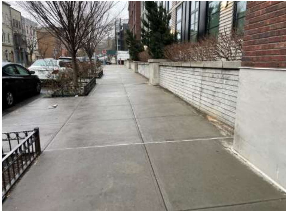
Photo 2: 2nd Street sidewalk, facing northwest. 02 March 2023.
