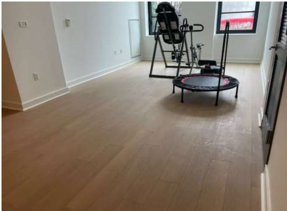
Photo 21: First floor concrete slab covered with wood within a typical residential tenant space, facing northeast. 02 March 2023.
