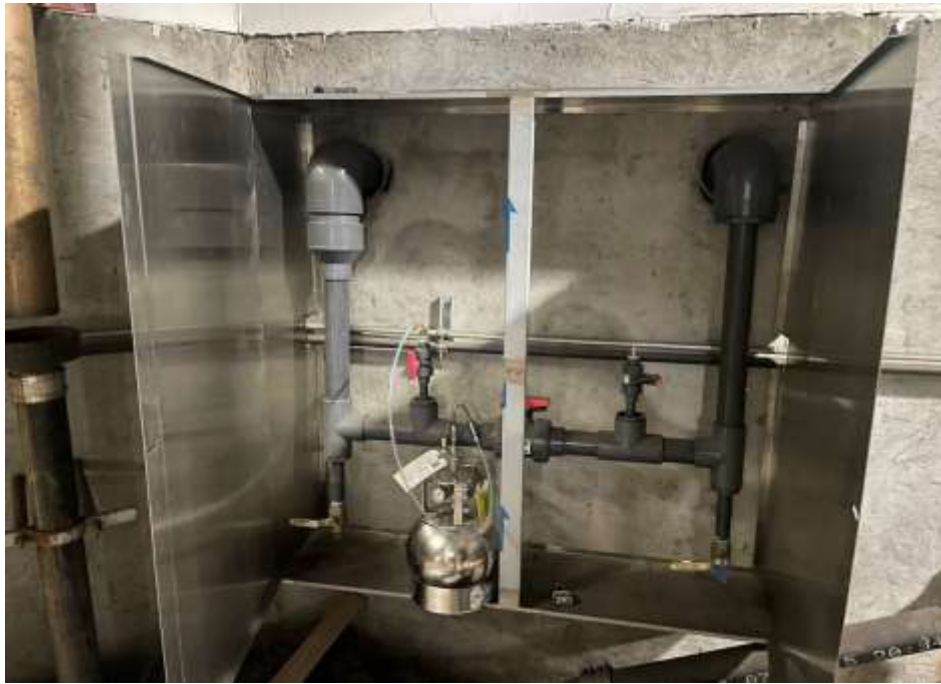
Photo 3: V2 subgrade sampling port in good condition, facing north. 05 December 2023.
