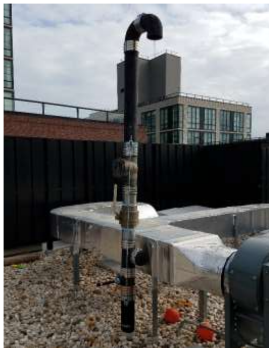
Photo 4: V3 riser in good condition, facing east. 20 June 2022.
