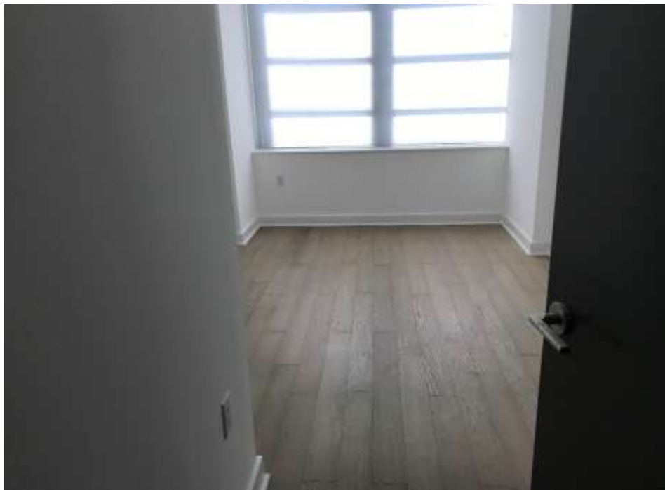
Photo 21: First floor concrete slab covered with wood within a typical residential tenant space, facing northeast. 20 June 2022.
