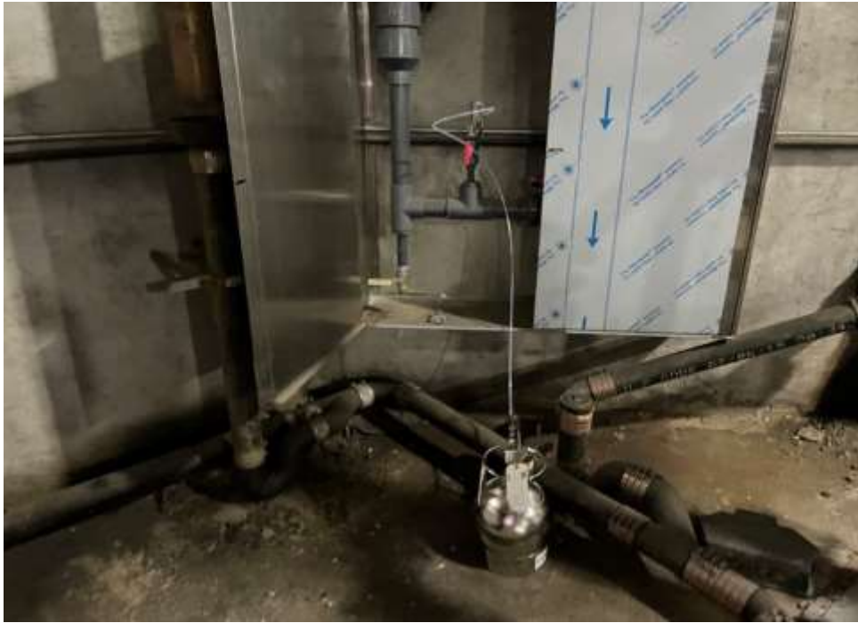
Photo 3: V2 subgrade sampling port in good condition, facing north. 20 June 2022.
