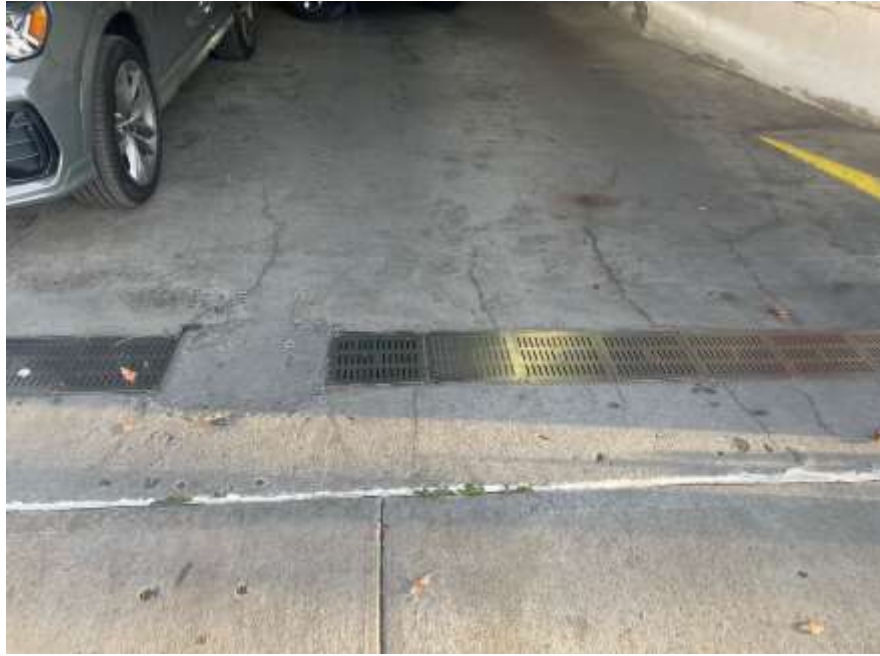
Photo 9: Typical hairline/surficial crack observed in the parking garage, facing north. Cracks did not breach to the subsurface. 02 March 2023.
