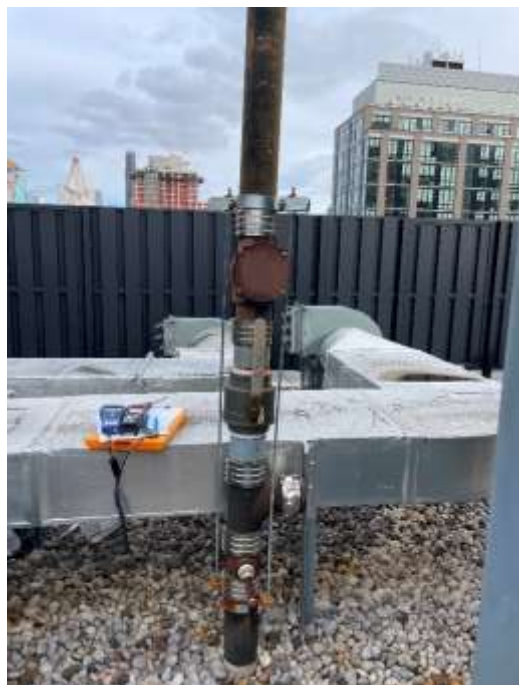
Photo 4: V3 riser in good condition, facing east. 02 March 2023.
