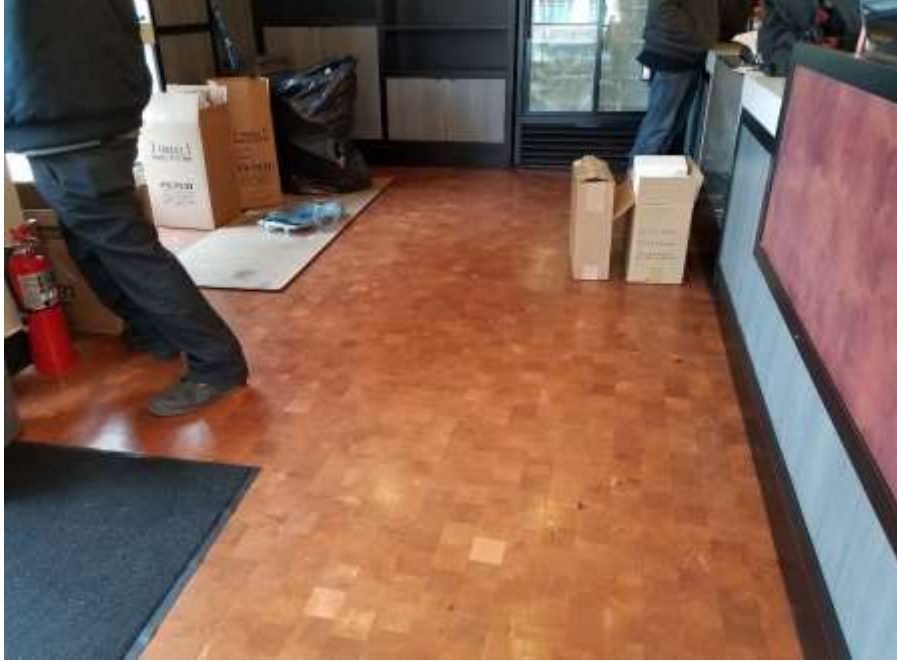
Photo 15: First floor concrete slab covered in tile flooring within the commercial space, facing northwest. 20 June 2022.
