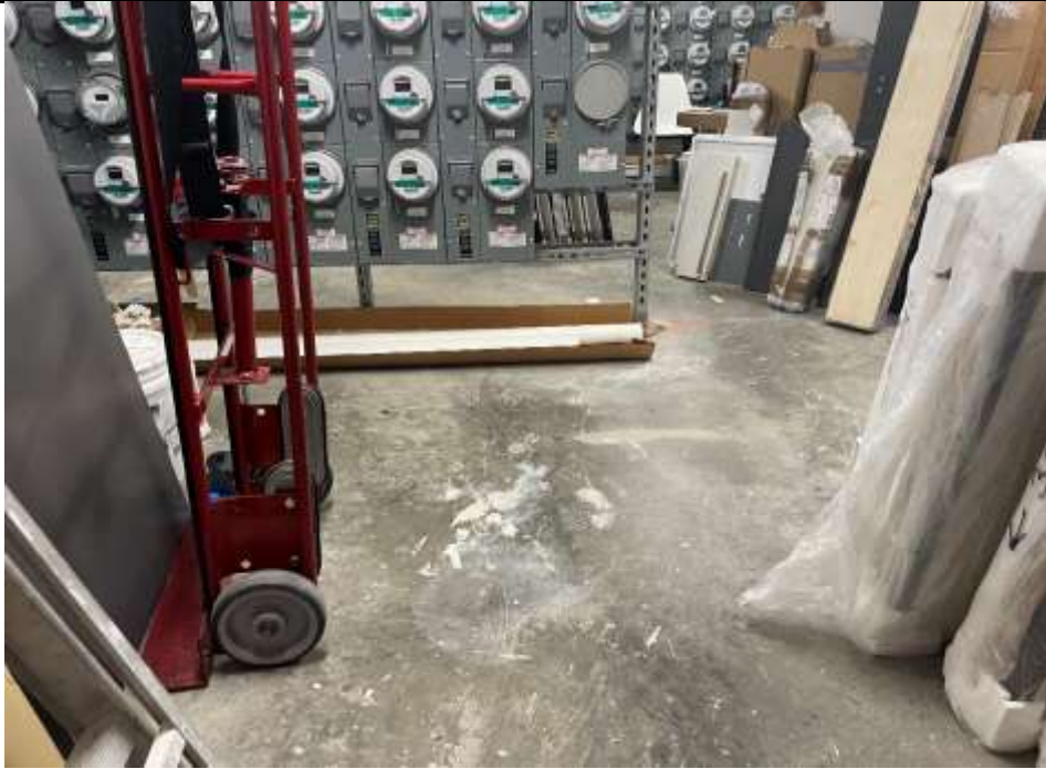
Photo 19: First floor concrete slab within the utility room, facing northeast. 02 March 2023.
