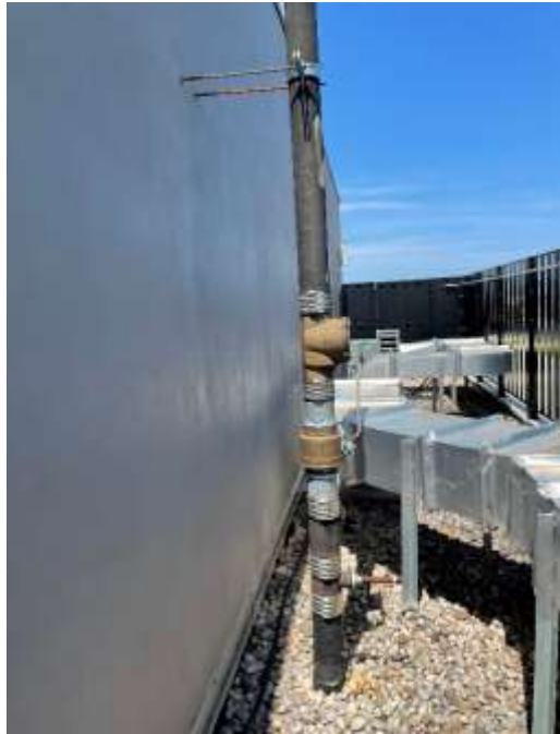
Photo 7: V4 riser in good condition, facing west. 20 June 2022.
