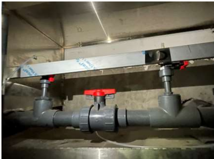
Photo 6: V3 subgrade sampling port in good condition, facing east. 02 March 2023.
