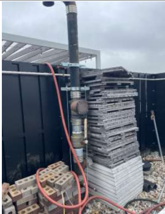
Photo 9: V5 riser in good condition, facing southeast. 02 March 2023.
