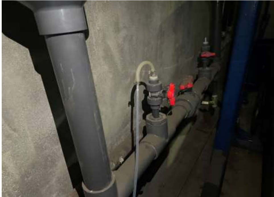
Photo 11: V5 subgrade sampling port in good condition, facing south. 02 March 2023.
