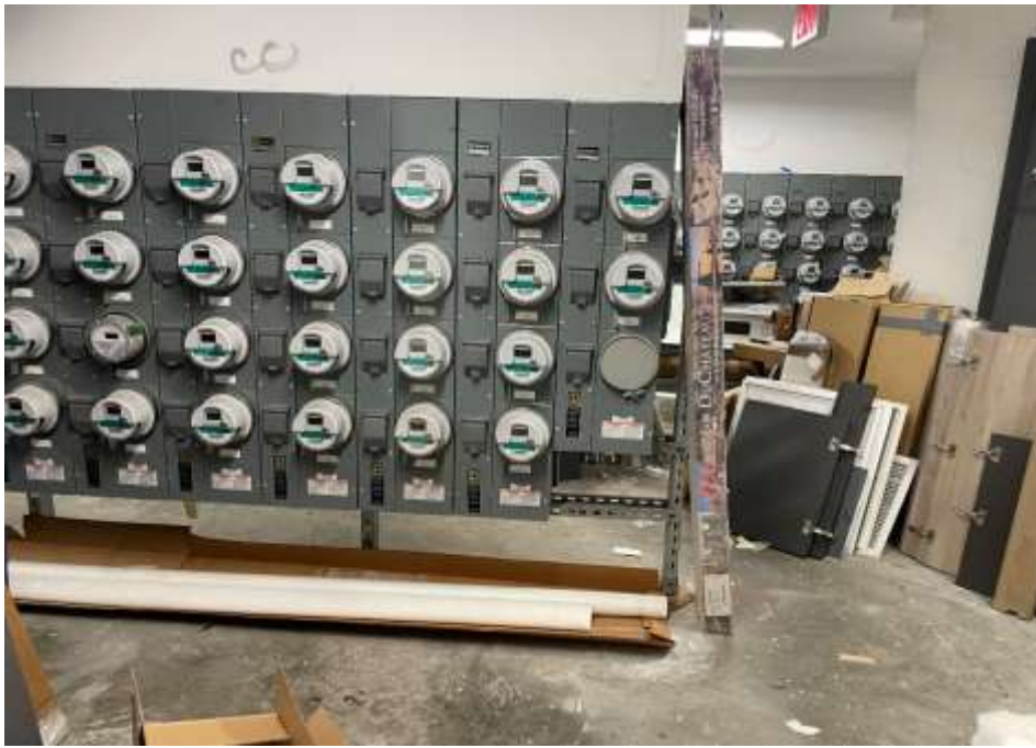
Photo 19: First floor concrete slab within the utility room, facing northeast. 05 December 2023.
