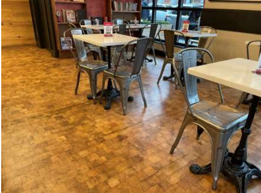
Photo 15: First floor concrete slab covered in tile flooring within the commercial space, facing northwest. 05 December 2023.
