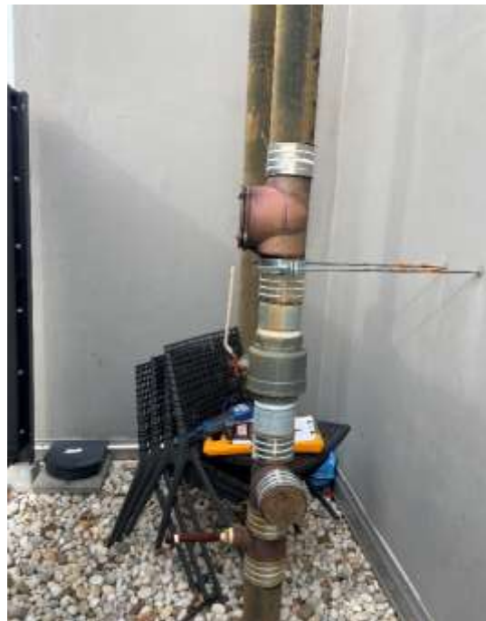
Photo 12: V6 riser and sample port in good condition, facing northwest. 05 December 2023.
