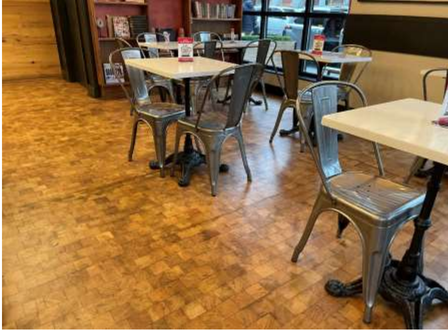
Photo 15: First floor concrete slab covered in tile flooring within the commercial space, facing northwest. 02 March 2023.
