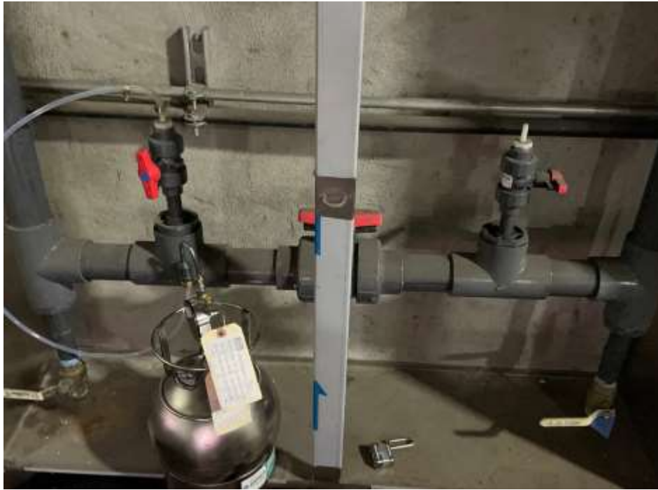
Photo 3: V2 subgrade sampling port in good condition, facing north. 02 March 2023.
