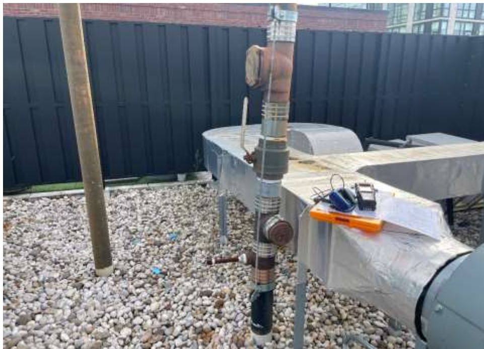
Photo 2: V1 riser and sample port in good condition, facing east. 05 December 2023.
