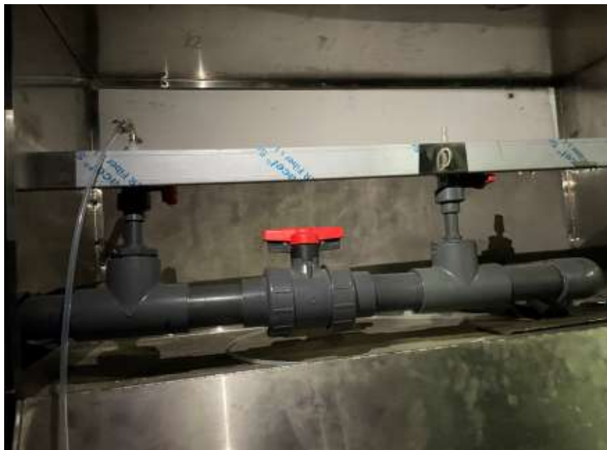
Photo 6: V3 subgrade sampling port in good condition, facing east. 20 June 2022.
