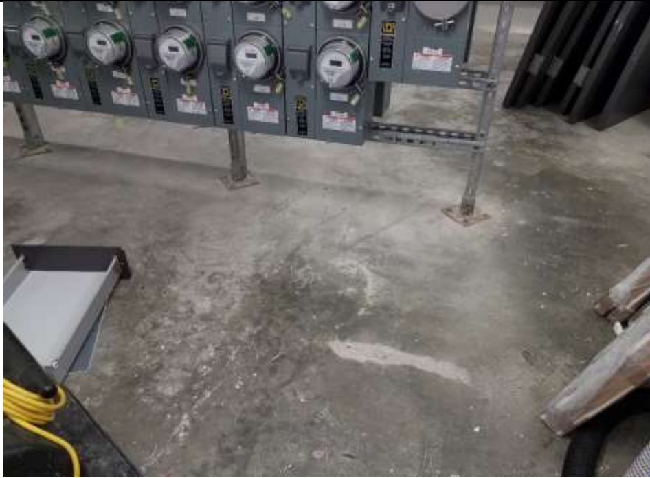
Photo 19: First floor concrete slab within the utility room, facing northeast. 20 June 2022.
