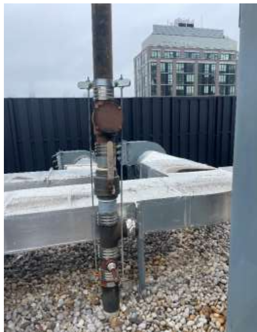
Photo 4: V3 riser in good condition, facing east. 02 March 2023.
