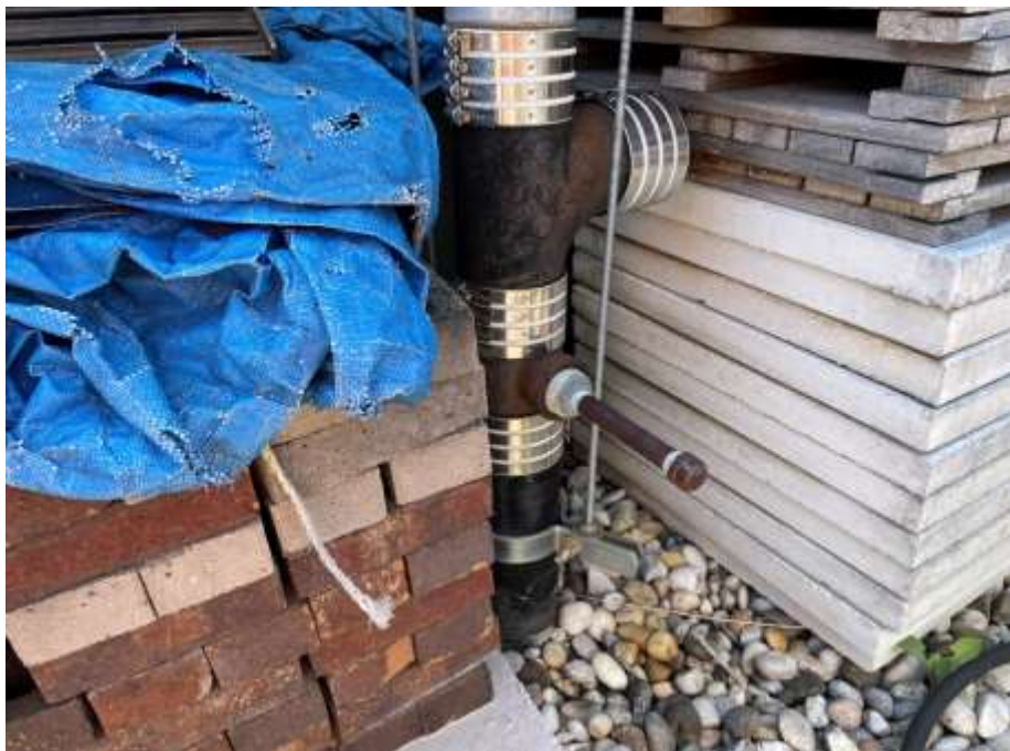
Photo 10: V5 riser and sample port in good condition, facing southeast. 20 June 2022.
