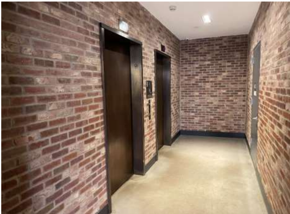
Photo 18: First floor concrete slab covered with flooring, facing west. 02 March 2023.
