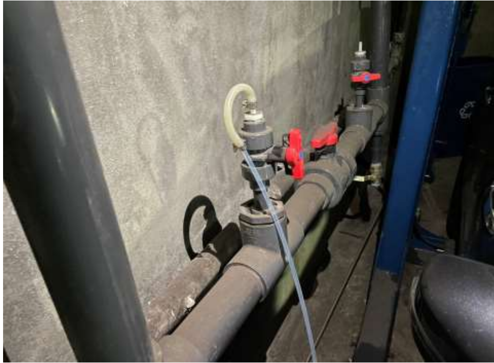
Photo 11: V5 subgrade sampling port in good condition, facing south. 02 March 2023.
