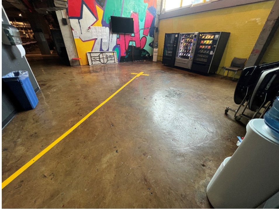
Photograph No. 7: Basement cover system consisting of epoxy sealed concrete floors.
