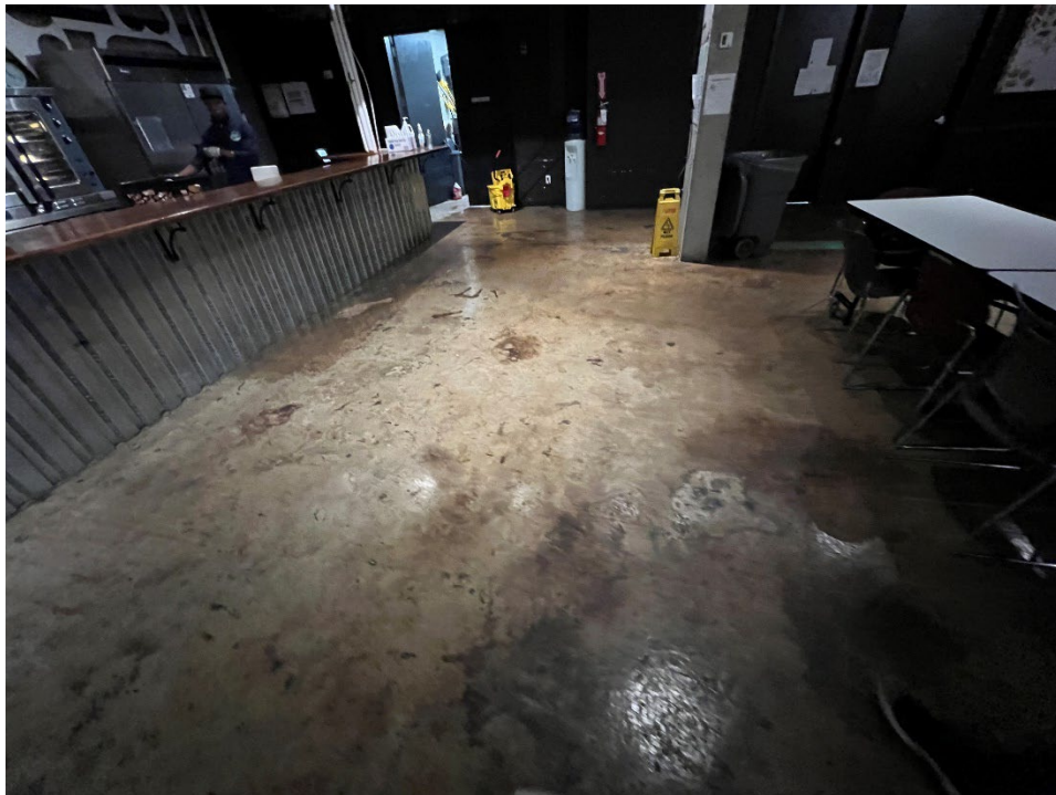
Photograph No. 6: Basement cover system consisting of epoxy sealed concrete floors.
