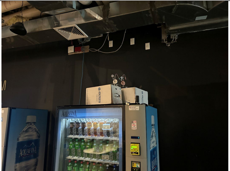
Photo 6 – View of the indoor air sample location IA-07, along with a duplicate sample, collected within the central portion of the cellar.
