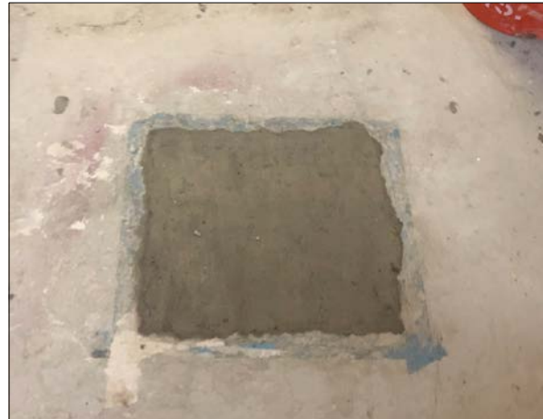
Pit after Filled with Concrete
