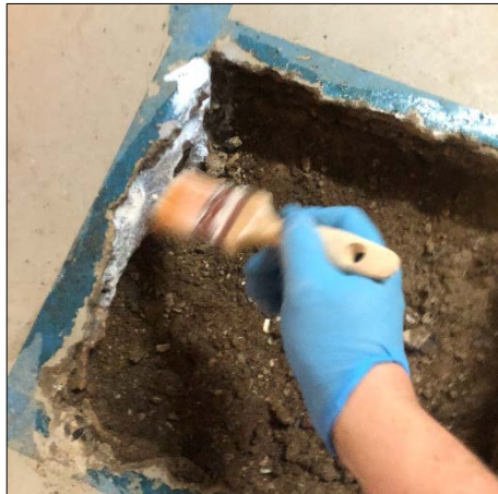
January 7, 2020 Photographs of Pit Closure: Application of Bonding Adhesive
