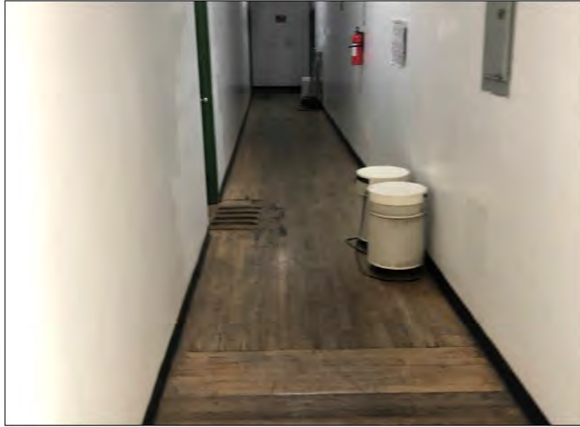
Photograph 9. Air filtration units in the second-floor central hallway.
