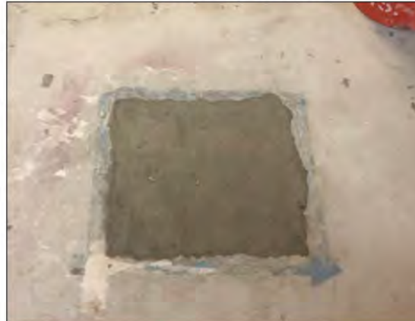
Pit after Filled with Concrete
