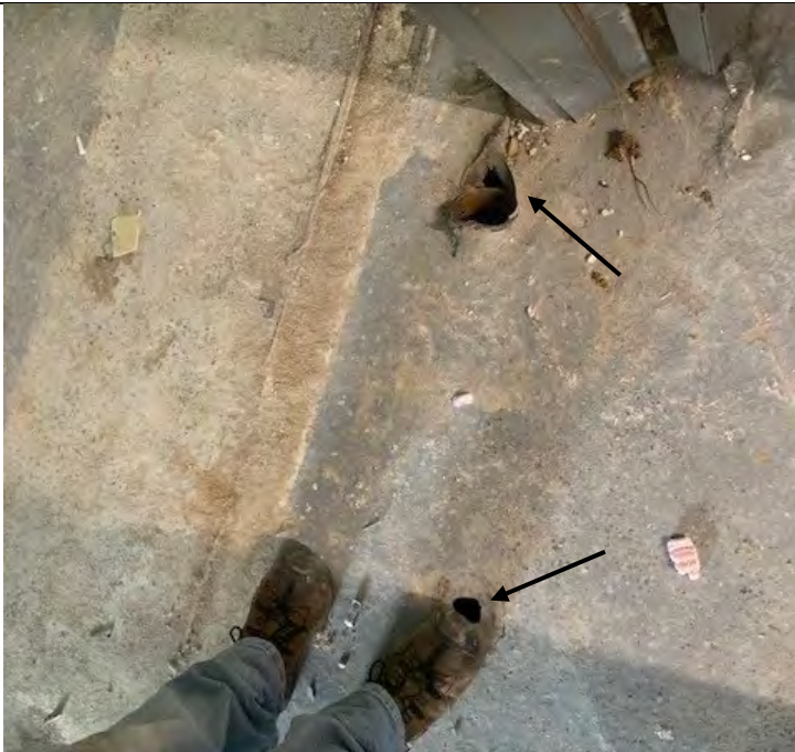
Photo 3. Pipe openings identified in former Blossom ice cream commercial space
