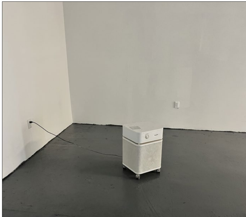
Photograph 8. Air filtration unit in a first-floor vacant section. December 8, 2022.
