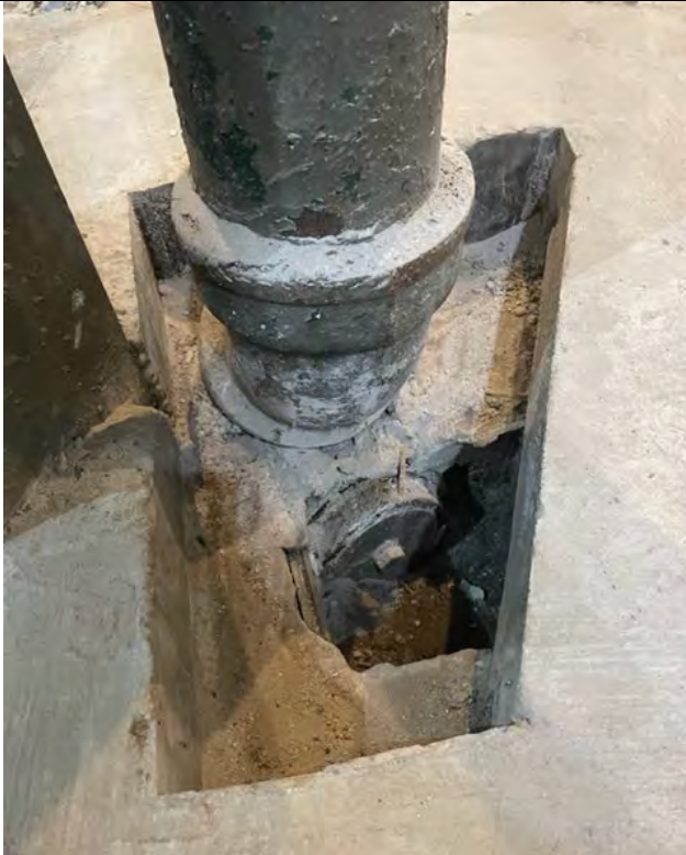
Photo 1. Slab cutout at base of vertical sewer pipe
