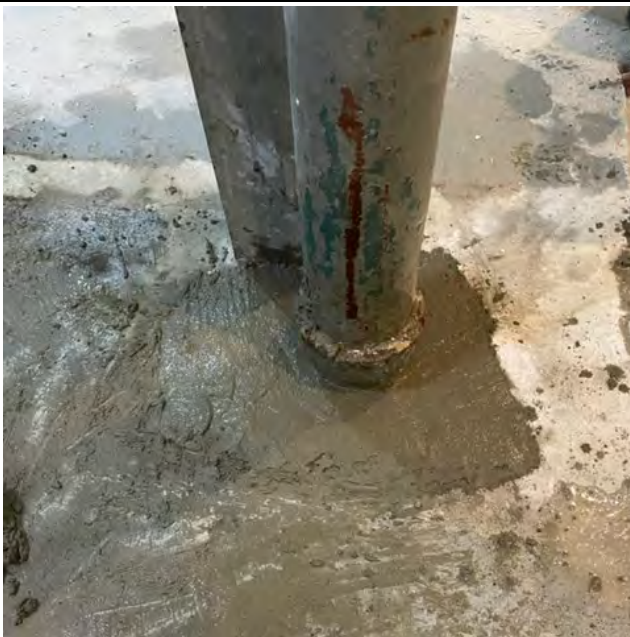
Photo 2. Slab cutout at base of vertical sewer pipe filled with concrete
