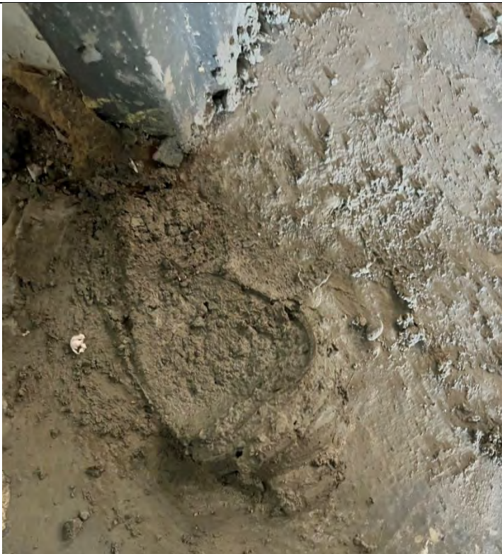
Photo 4. Concrete filling pipe opening shown in upper portion of Photo 3
