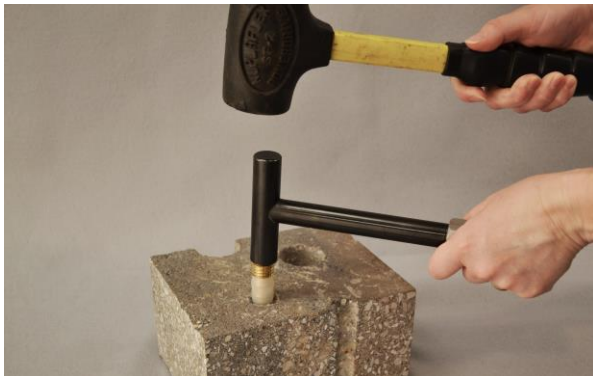
Figure 2. Installing the VAPOR PIN®
