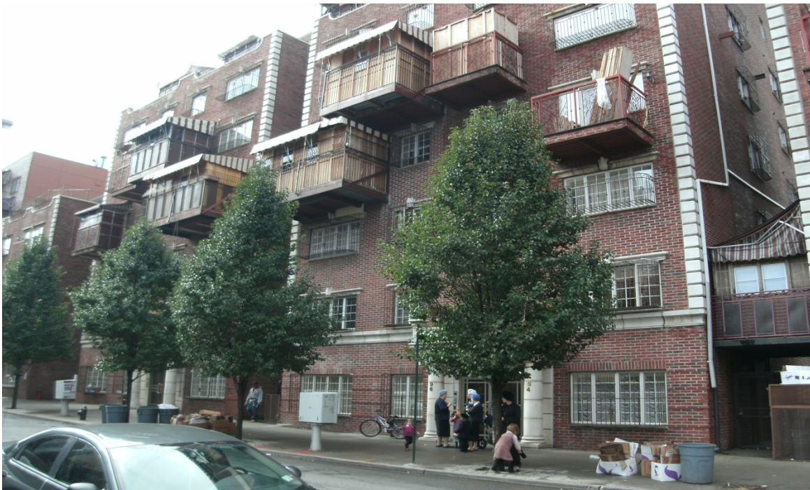
View of the western adjacent properties, looking southwest across Skillman Street.
