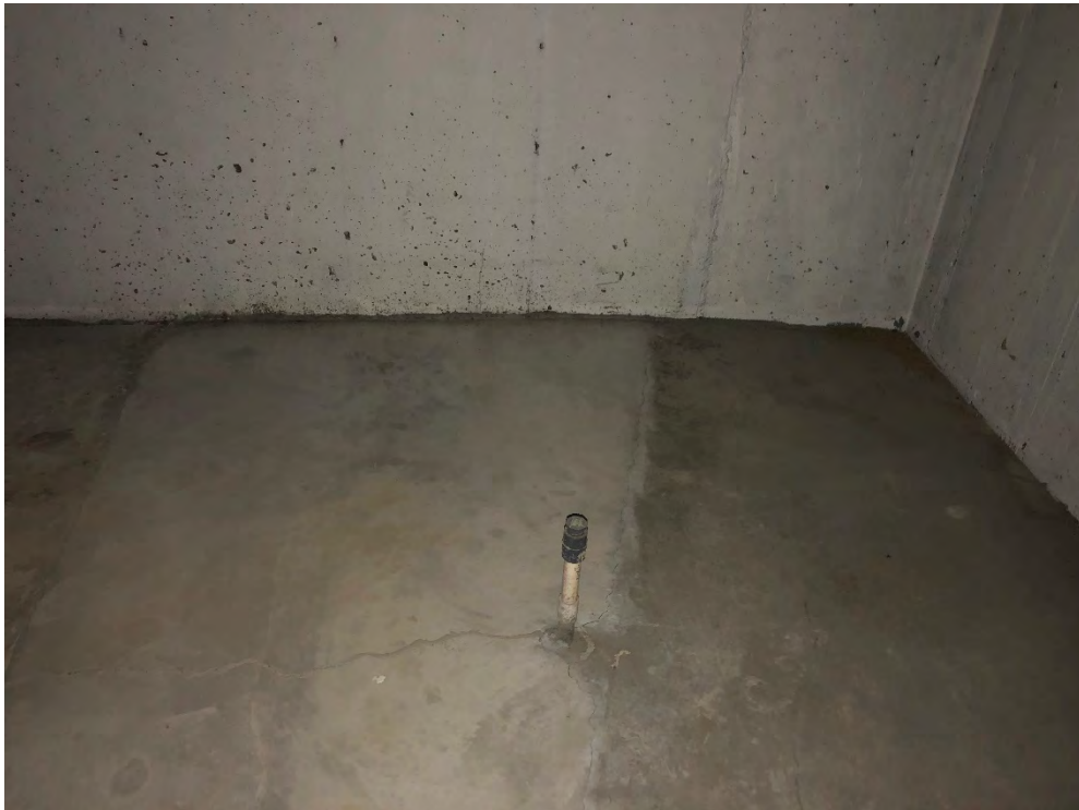
Photo 6: Photo of the northeast corner in the northern basement.
