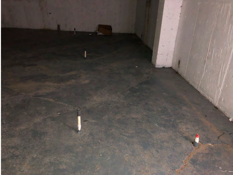
Photo 5: Representative photo of the southern basement (looking north); injection points and MW-1 are in view.
