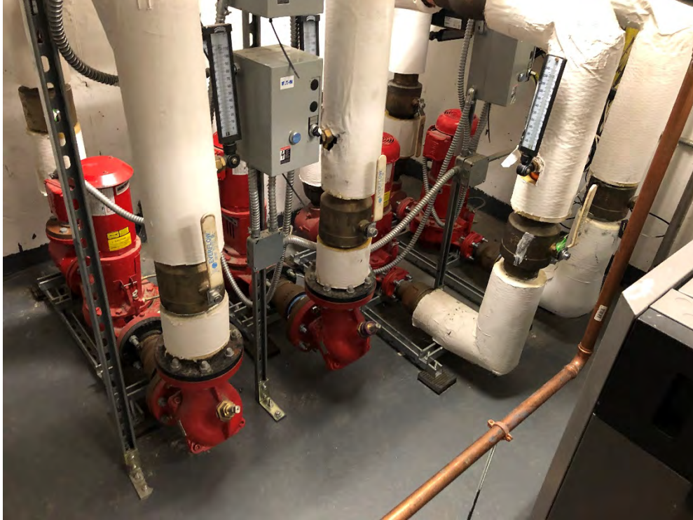
Photo 3: Photo of the concrete slab in the Site's boiler room (southeast corner).
