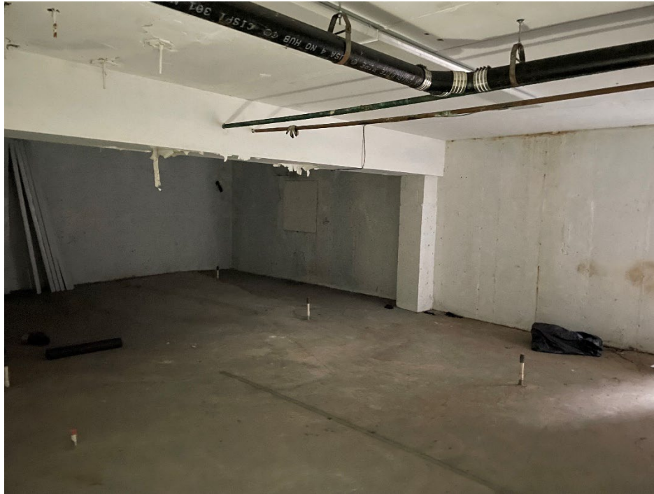
Photo 13: Photo showing intact concrete composite cover system located in the southern commercial space basement.
