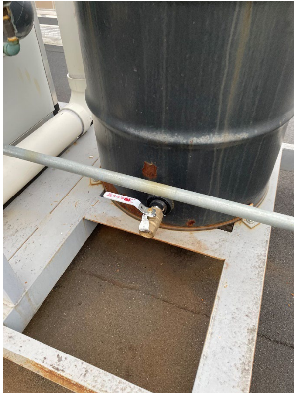
Photo 6: Photo of checking Blower A knockout tank during the inspection. Tank was found to be empty.
