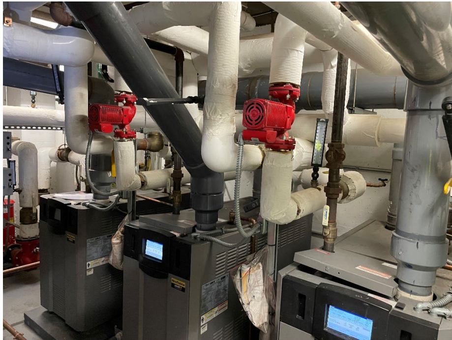
Photo 18: Inspection of the boiler room piping and foundation.
