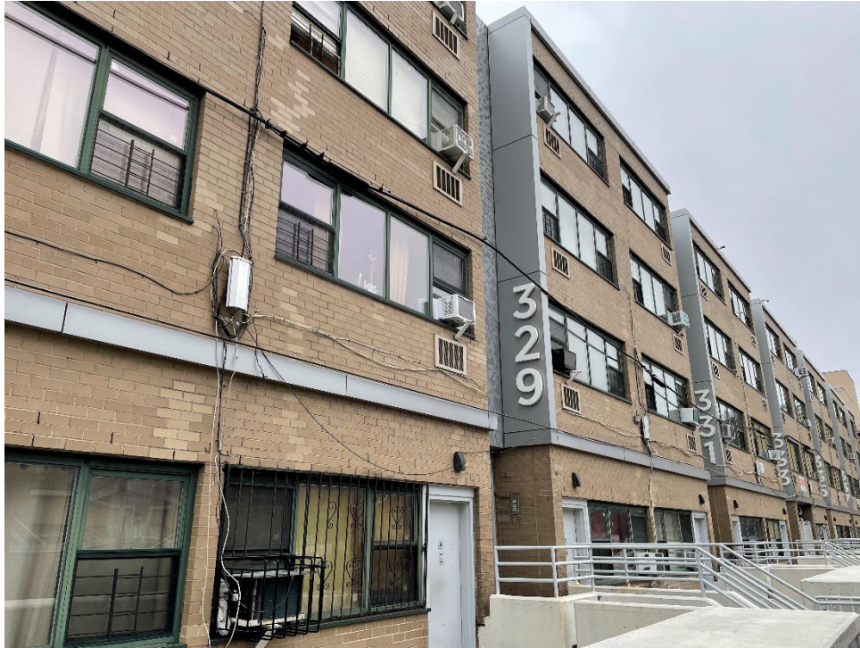
Photo 15: Looking south, showing residential side of the site and stairwells leading to basements where SVMP's are located.
