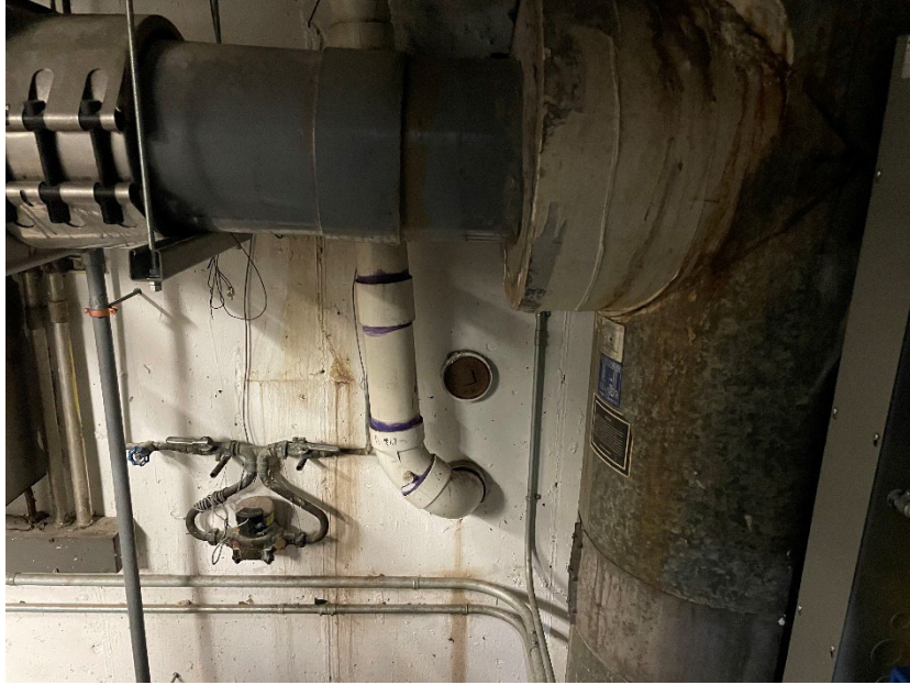
Photo 9: Looking south, view of monitoring point SVMP-A2 in the boiler room and SSDS leg going into the wall.
