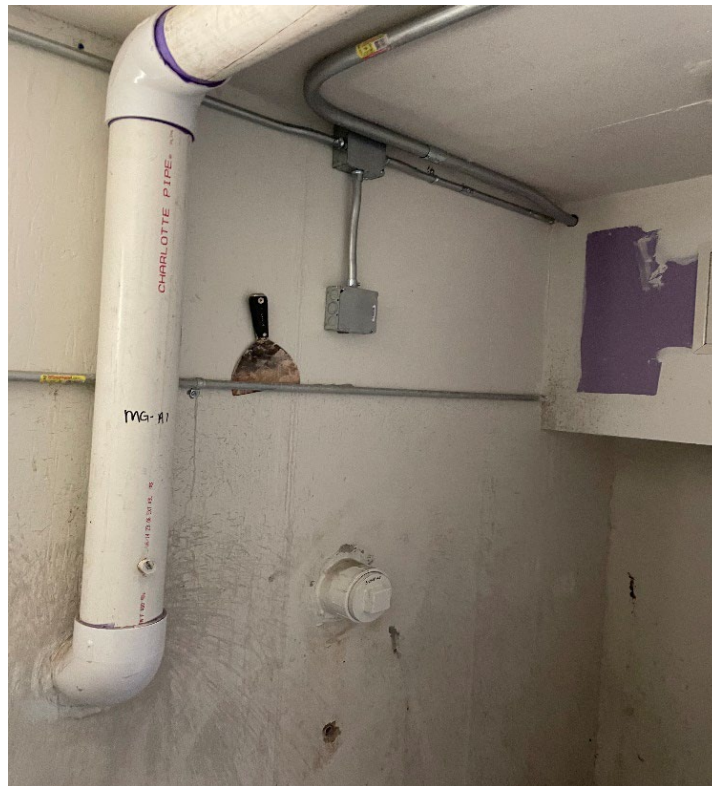
Photo 10: Photo of SVMP-A5 during annual inspection with adjacent suction point MG-A1. The suction point showed significant a vacuum measurement during inspection (Appendix F).
