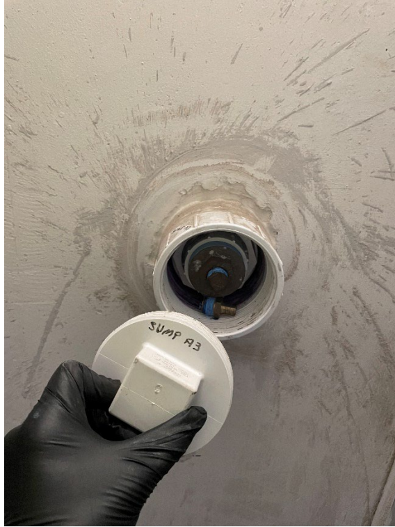
Photo 19: Photo showing monitoring point SVMP-A3 located on the residential side of the site.
