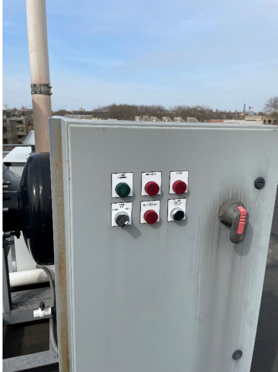
Photo 3: View of Blower B (northern) SSDS control panel.
