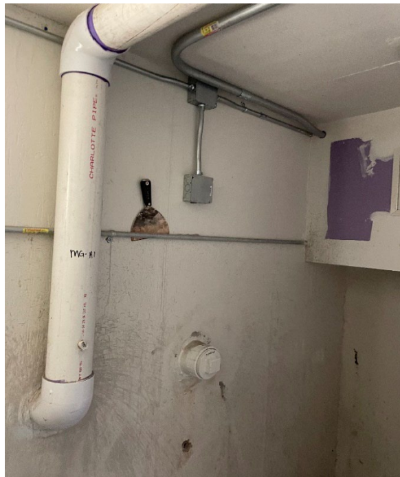
Photo 10: Photo of SVMP-A5 during annual inspection with adjacent suction point MG-A1. The suction point showed significant a vacuum measurement during inspection (Appendix F).
