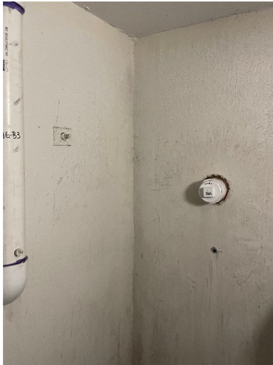
Photo 16: Photo showing monitoring point SVMP-B4 and suction point MG-B3 during site inspection.
