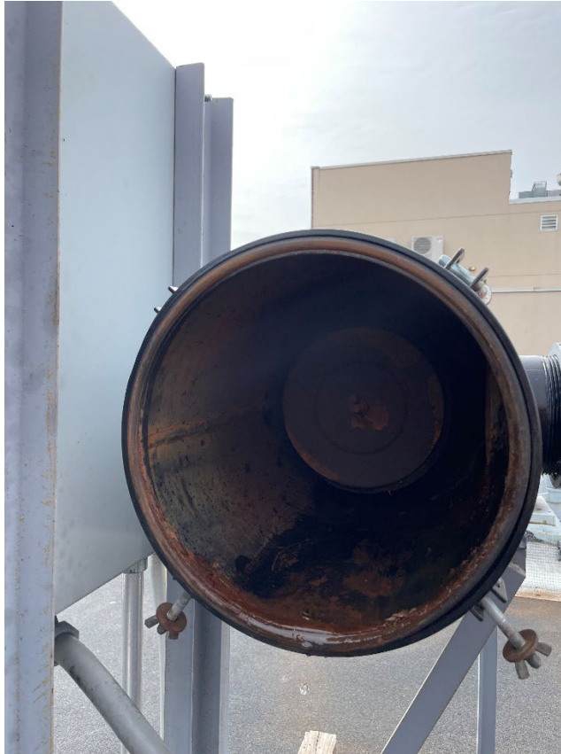
Photo 19: Photo during inspection and replacement of the air intake filter.
