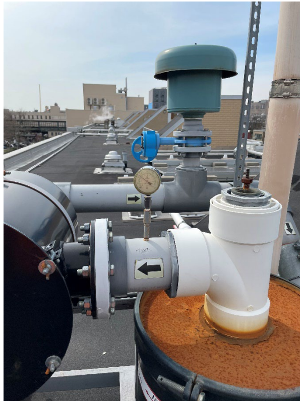
Photo 6: Photo of knockout/condensate tank influent gauge on the Blower B unit.
