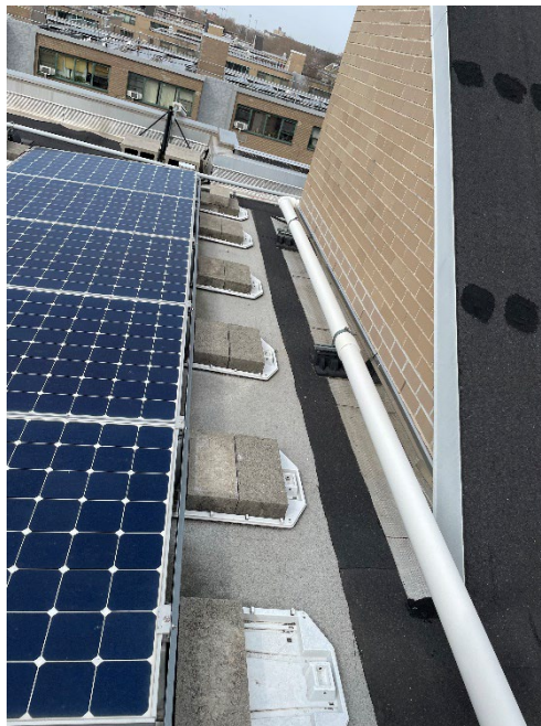
Photo 8: Looking west, photo showing SSDS piping run along the roof with legs leading towards the residential building side.
