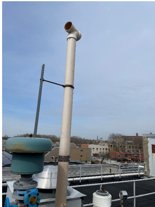
Photo 4: View of Blower B discharge stack.
