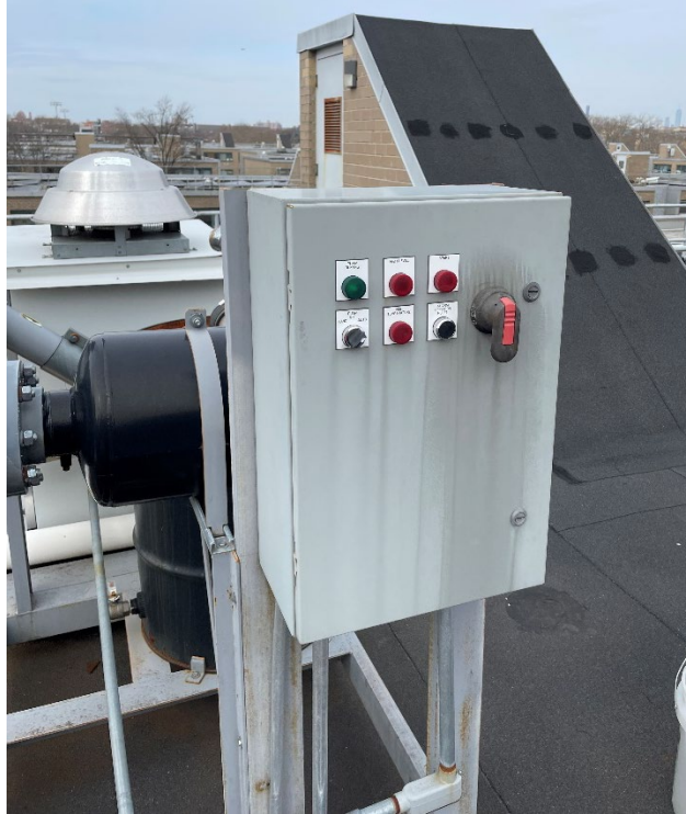
Photo 1: View of Blower A (southern) SSDS control panel with functioning “pump running” bulb shown as functional.
