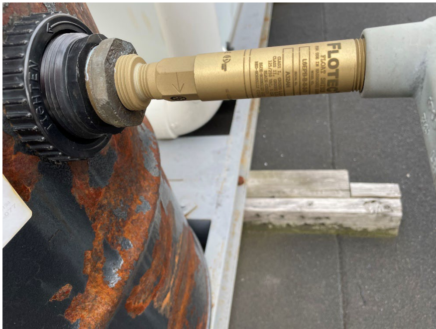
Photo 2: View of new float switch that was installed as part of the routine maintenance performed on Blower A throughout the reporting period.
