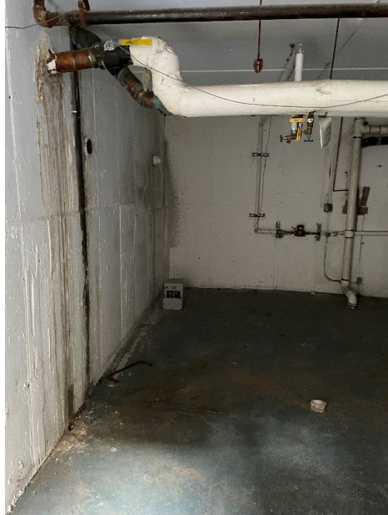
Photo 11: Looking west, view of SSDS legs belonging to the Building B blower (southern basement area); SVMP-B3 is located on the south wall.
