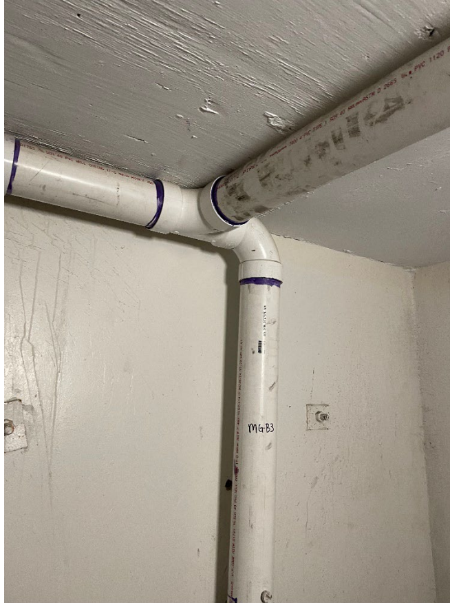
Photo 17: Photo showing suction point MG-B3 leg distribution.
