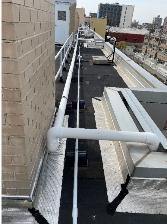
Photo 7: Looking south, photo showing SSDS piping run along the roof with legs heading down the residential side of the building.
