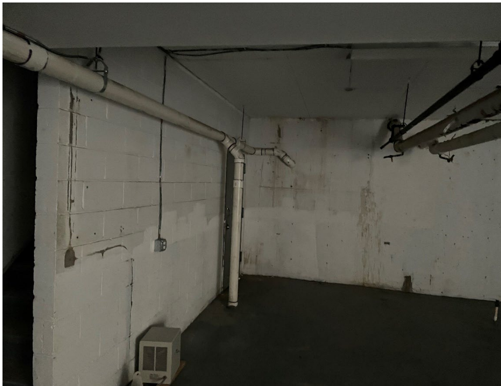
Photo 12: Photo of the southern basement located under the commercial spaces; network of legs and suction points MG10 through MG-12.
