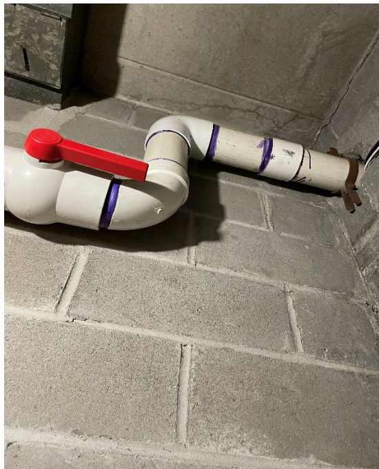
Photo 20: SSDS piping run leading down from the first floor and into the boiler room wall; valve is in the full open position.
