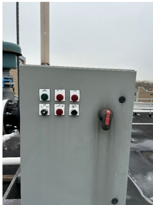
Photo 2: View of Blower B (northern) SSDS control panel.
