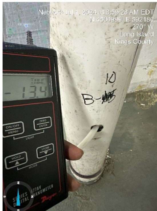
Photo 28: Photo of manometer reading of suction point MG-B10
