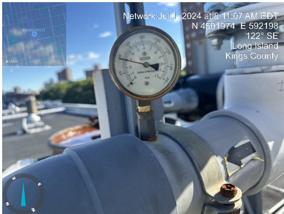
Photo 26: Photo of the gauge on the Blower unit
