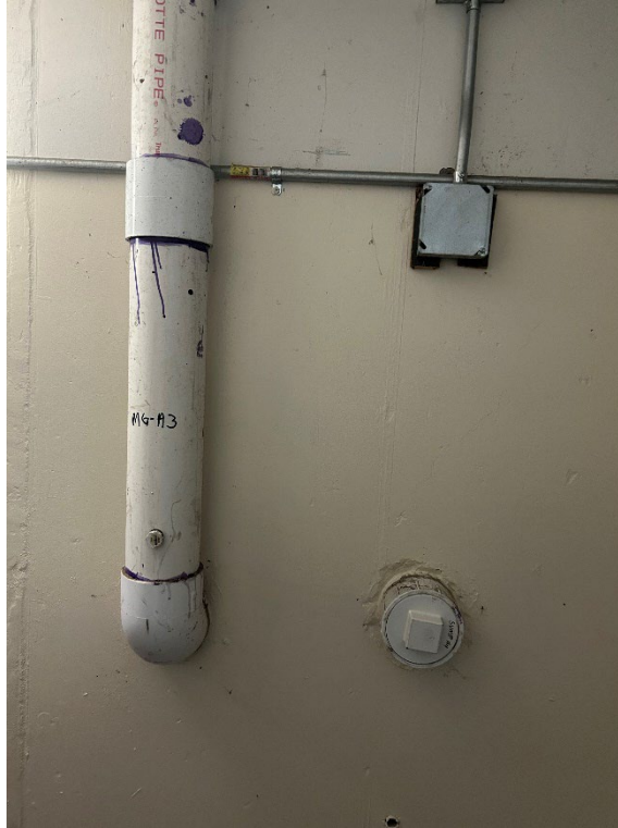
Photo 9: Photo of SVMP-A4 during annual inspection with adjacent suction point MG-A3.
