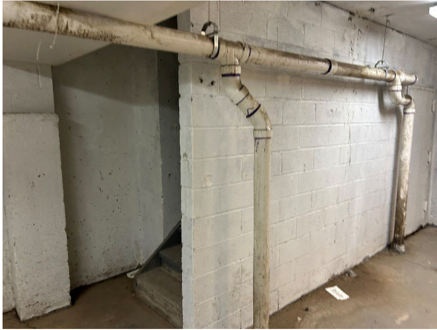
Photo 19: Photo of the southern basement located under the commercial spaces; network of legs and suction points and of one of the basement staircases.
