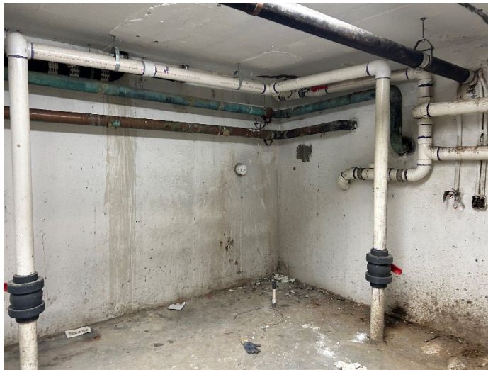
Photo 18: Photo of the southern basement located under the commercial spaces; network of legs and suction points.
