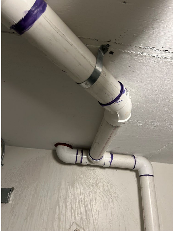
Photo 17: Photo showing suction point MG-B7 leg distribution.
