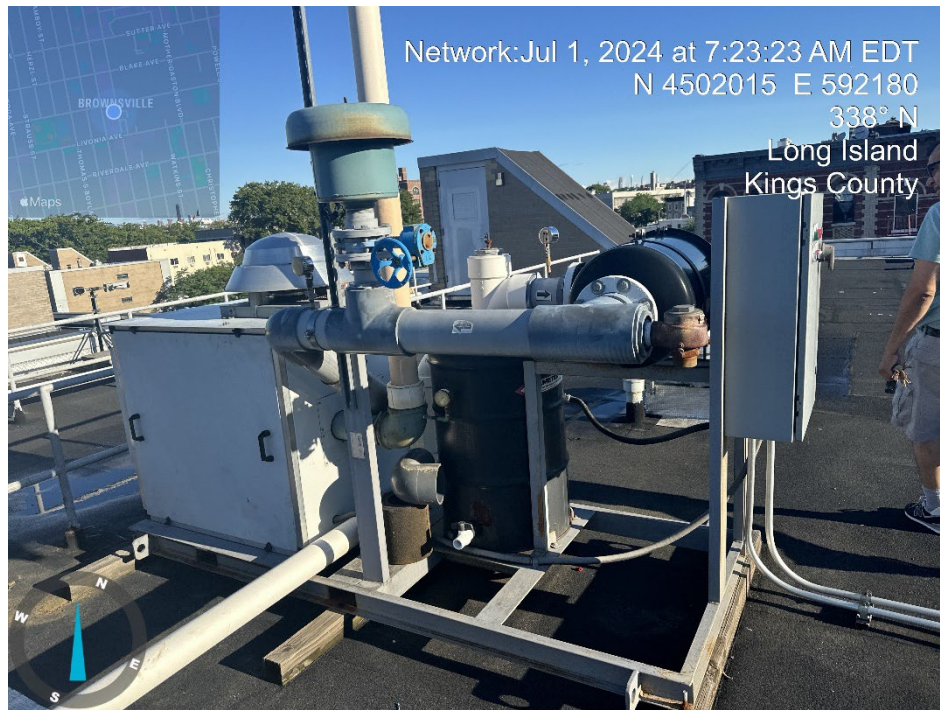
Photo 21: Overview of SSDS Blower B after maintenance and re-start.
