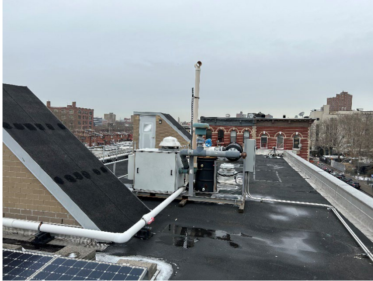
Photo 3: View of Blower B discharge stack.
