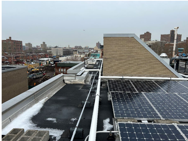
Photo 6: View showing SSDS piping run along the roof with legs heading down the side of the building.
