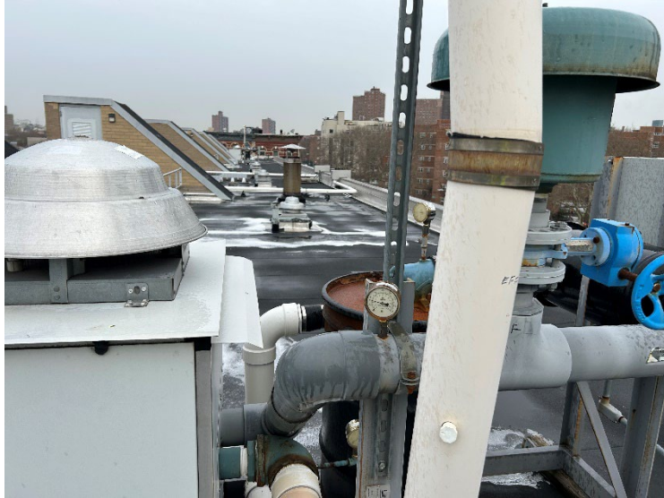
Photo 5: Photo of inlet gauge and piping at Blower B.
