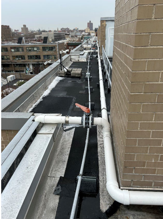
Photo 7: View showing SSDS piping run along the roof with legs heading down the side of the building.
