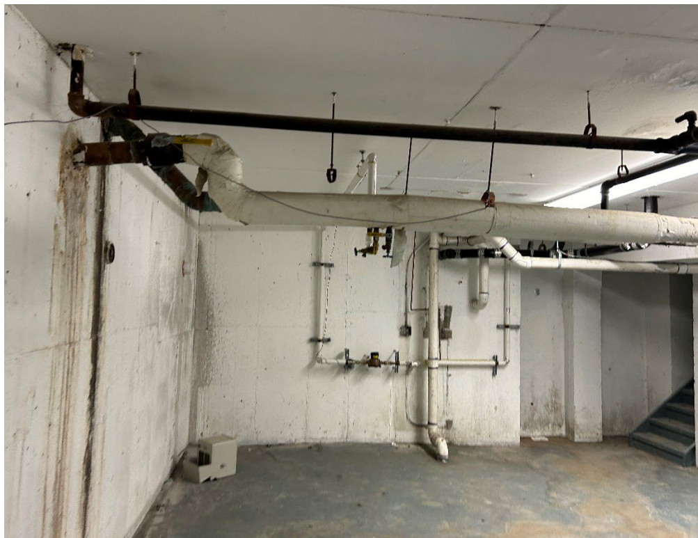
Photo 12: : Looking west, view of SSDS legs belonging to the Building B blower (southern basement area); SVMP-B3 is located on the south wall.
