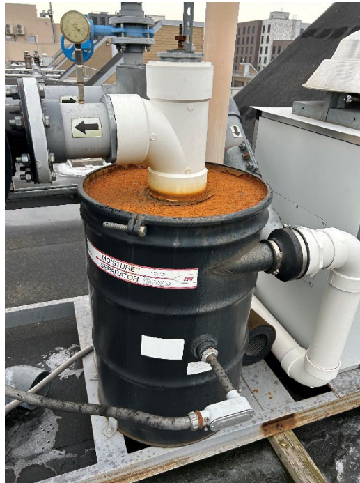
Photo 4: Photo of knockout/condensate tank influent gauge on the Blower B unit.
