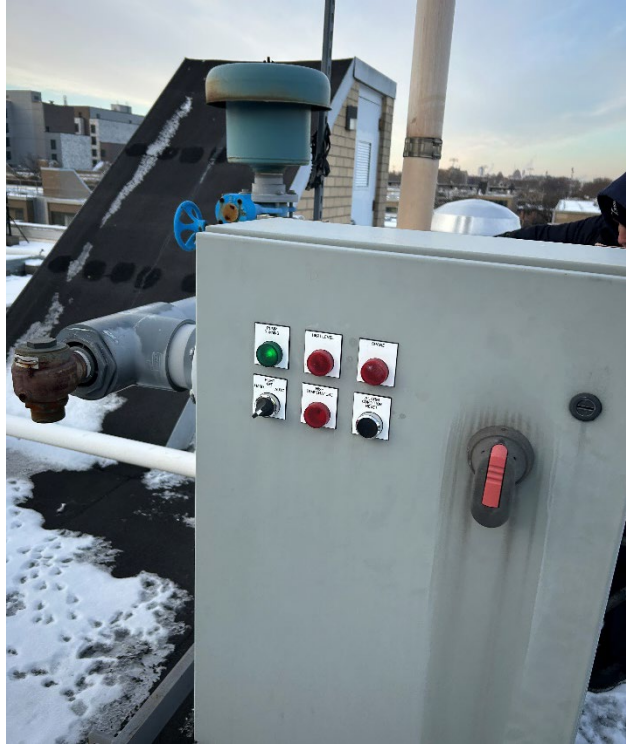
Photo 1: View of Blower B (northern) SSDS control panel with functioning “pump running” bulb shown as functional.
