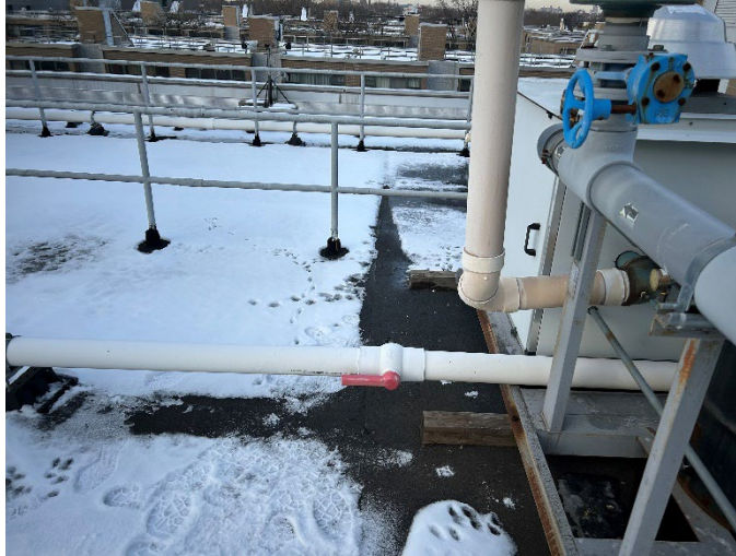
Photo 13: SSDS piping run along the roof from Blower A; valve is in the full open position.
