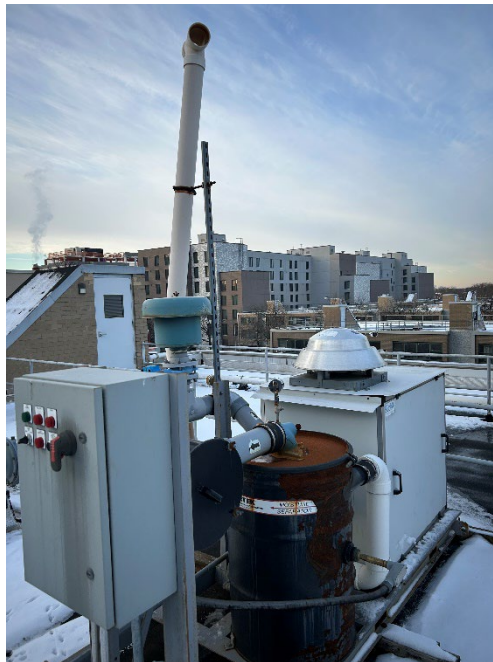
Photo 2: Overview of Blower A (southern) SSDS control panel and discharge stack.
