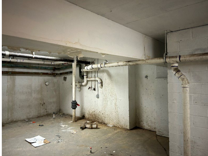
Photo 11: Photo of the southern basement located under the commercial spaces; network of legs and suction points.
