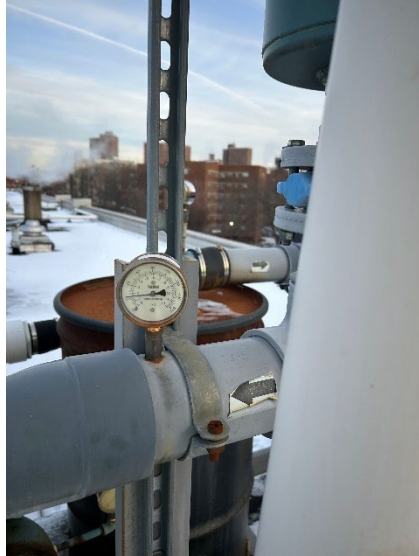
Photo 5: Photo of inlet gauge at Blower A.
