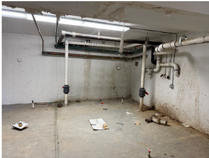
Photo 8: Photo of SVMP-B2 during annual inspection.
