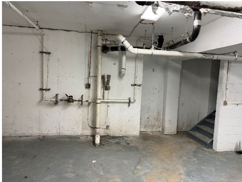
Photo 12: Photo of the southern basement located under the commercial spaces; network of legs and suction points and of one of the basement staircases.
