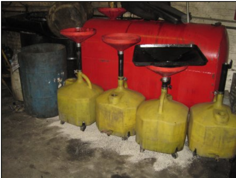
View of 275-gallon AST and additional oil containers along with staining within 262 Van Brunt Street.
