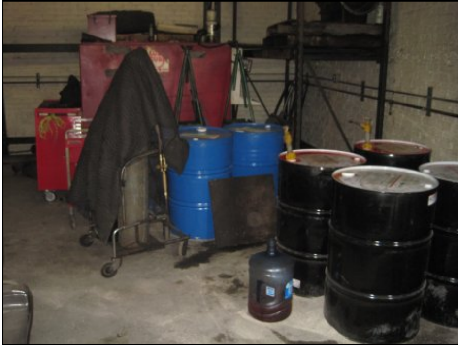
View of out-of-service 750-gallon AST and additional oil stored within drums.
