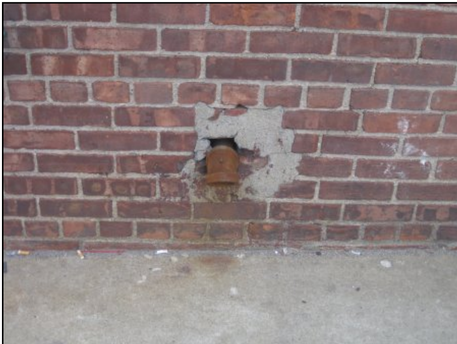
View of suspect former fuel oil vent pipe along 260 Van Brunt Street.
