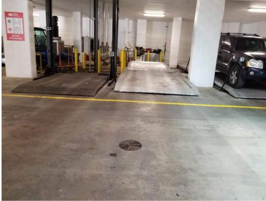
**Photograph 3:** Example car stackers and floor drain in the cellar level ventilated parking garage (03/29/2021)
