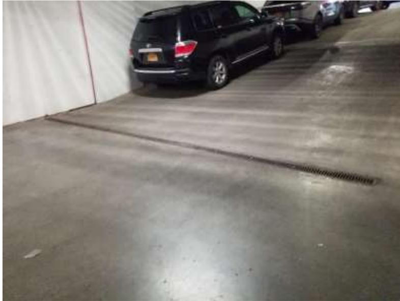
**Photograph 5:** View of example trench drain located within the cellar level ventilated parking garage (03/31/2022)
