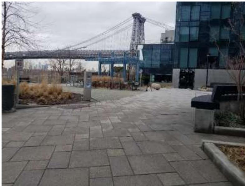
**Photograph 10:** View of composite cover including vegetation, concrete pavers, and gravel paved area installed within the esplanade in June 2021, facing northwest (03/31/2022)
