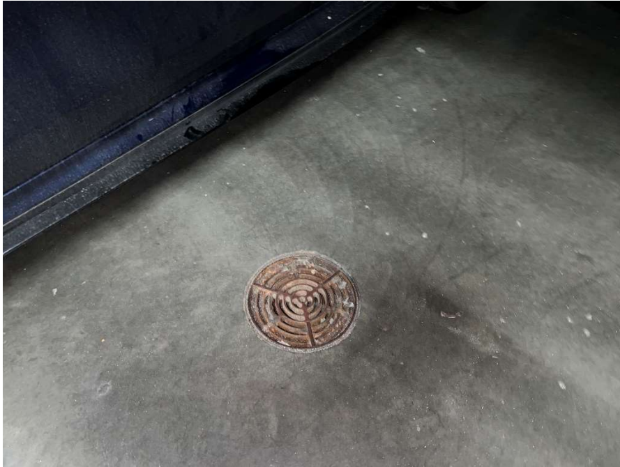
Photograph 3: Example floor drain in the cellar level ventilated parking garage (04/06/2023)
