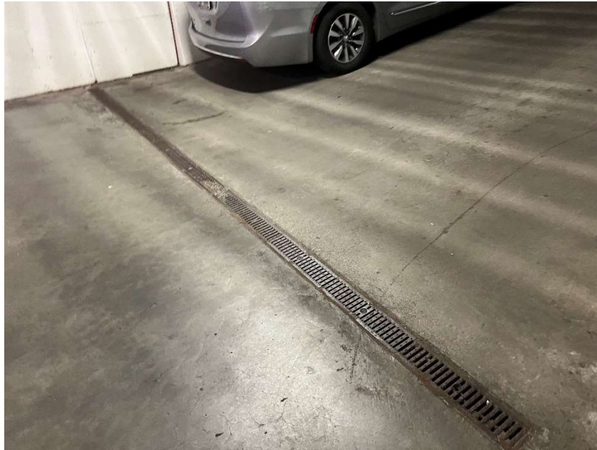
Photograph 5: View of example trench drain located within the cellar level ventilated parking garage (04/06/2023)
