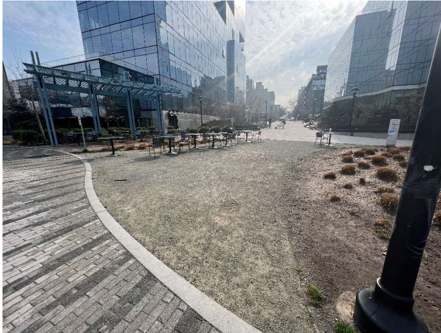
Photograph 9: View of composite cover including concrete pavers, stone dust, and vegetation near the southwestern corner of the 416 Kent building, facing east (04/06/2023)
