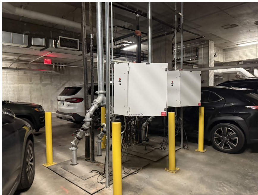
Photograph 4: View of sewer lift system/sump pits and pump located in the cellar level ventilated parking garage (03/28/2025)
