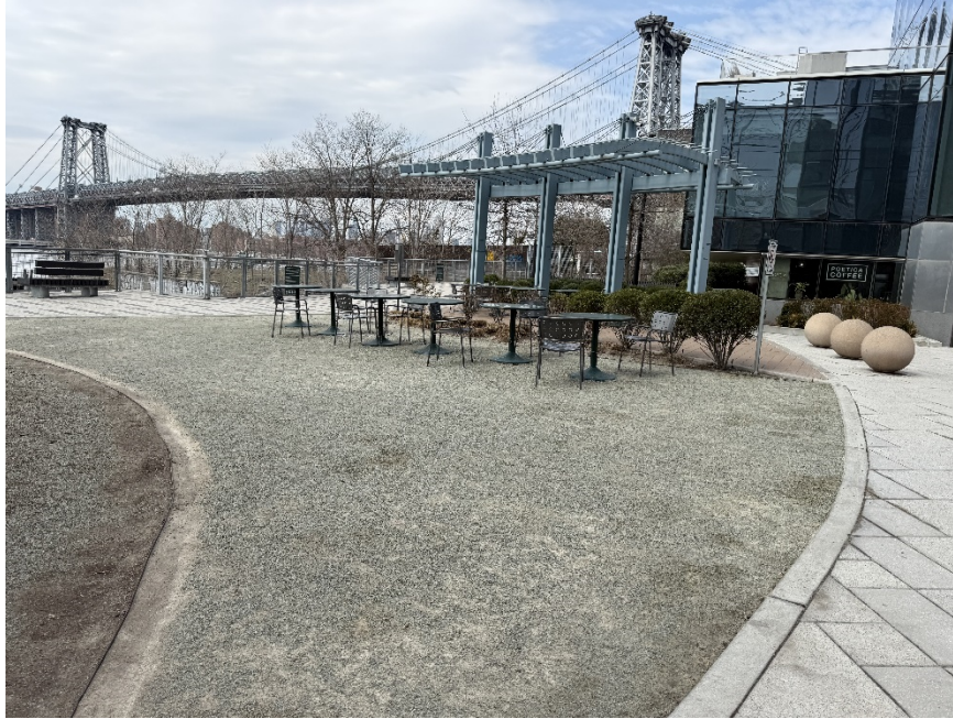
Photograph 9: View of composite cover including concrete pavers, stone dust, and vegetation near the southwestern corner of the 416 Kent building, facing north (03/28/2025)
