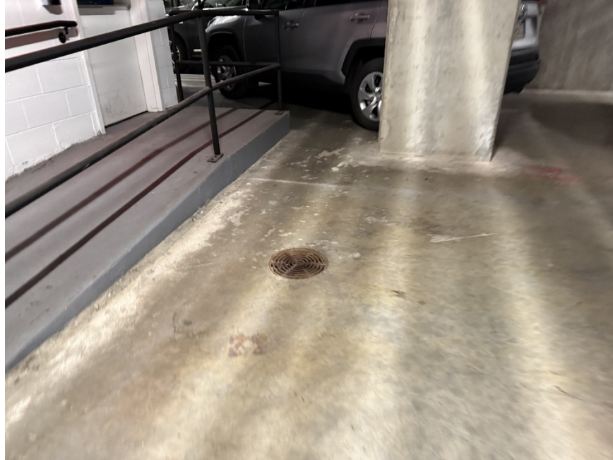
Photograph 3: Example floor drain in the cellar level ventilated parking garage (03/28/2025)
