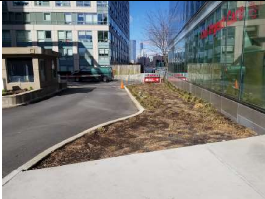
Photograph 11: View of the subsurface parking garage entrance located in the southeastern site corner, facing west (03/29/2021)
