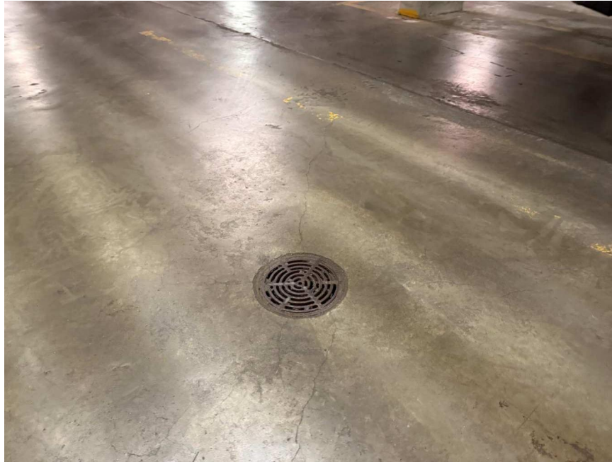
Photograph 5: Example floor drain in the cellar level ventilated parking garage (03/28/2025)
