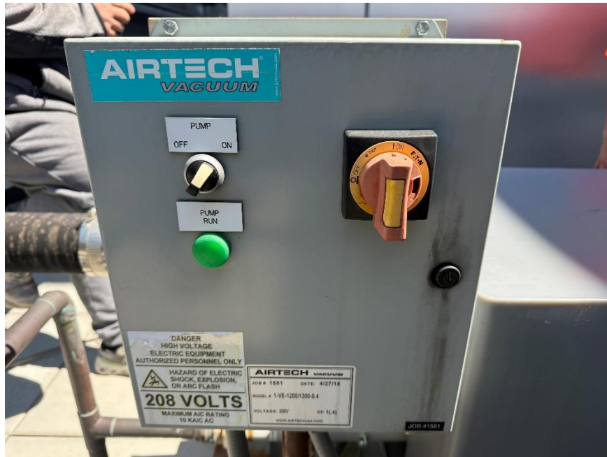
Photograph 6: View of blower box on the roof of the building, facing west (04/14/2026)
