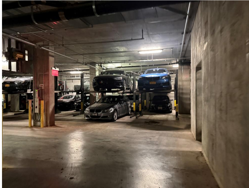
Photograph 5: Example view of car stackers in the cellar level ventilated parking garage (04/14/2026)
