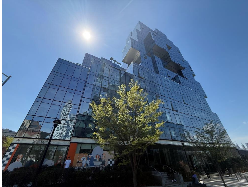
Photograph 1: View of 420 Kent from Kent Avenue (04/14/2026)
