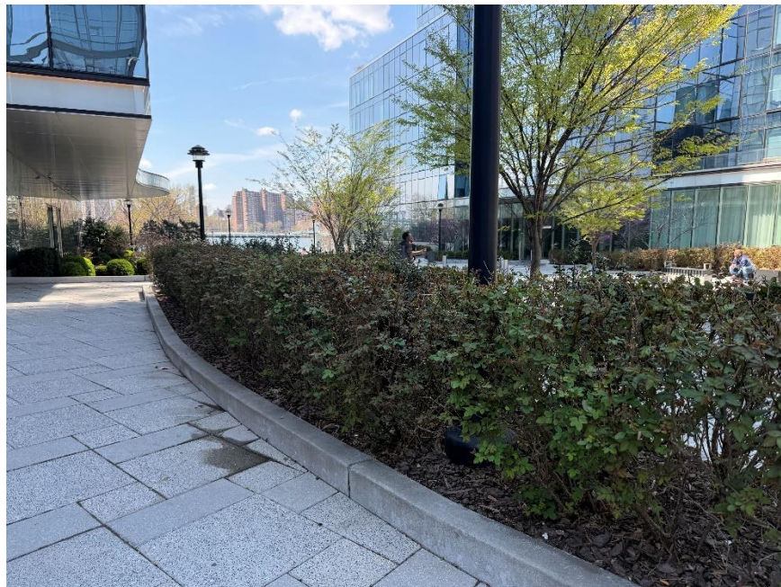
Photograph 12: View of the composite cover located in the northern part of the site (04/14/2026)
