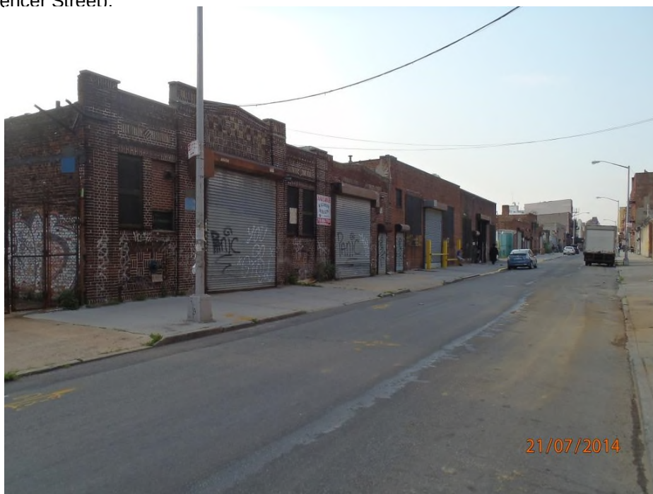
Photograph 2: View of the main cluster of Site buildings looking south along Spencer Street.
