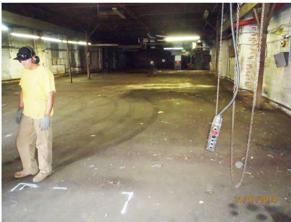
Photograph 6: General interior view of the former sheet metal manufacturing building looking south from the Flushing Avenue entrance. The white painted outline at lower left denotes subsurface anomaly resembling a UST.
