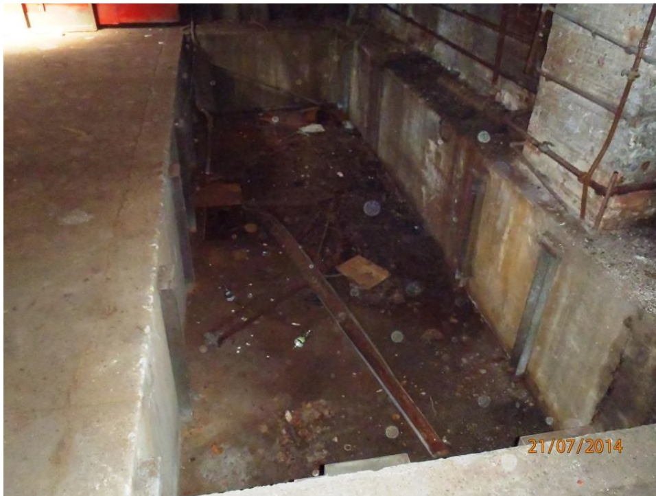
Photograph 5: Concrete pit within the former sheet metal manufacturing building.
