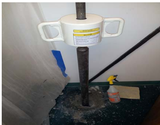
Photo 1: View of Geoprobe slide hammer utilized to collected sub-slab soil samples.
