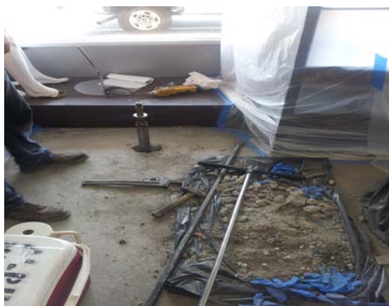
Photo 2: View of Geoprobe slide hammer beneath slab in GK Jeans unit.
