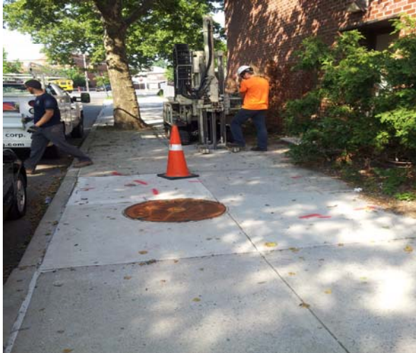
Photo 7: Soil Boring/Well installation.
