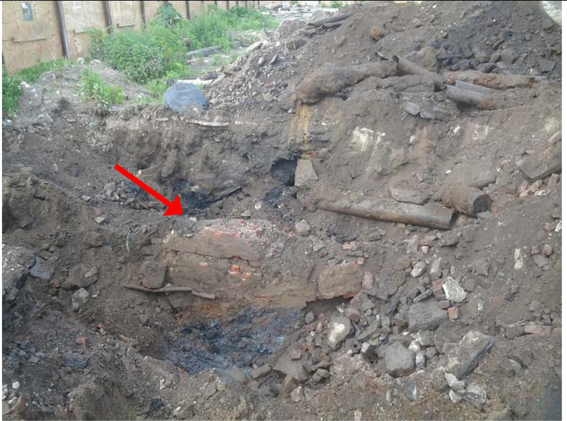
**Photo 4 – Several 8 to 12 inch diameter metal pipes were present in the utility tunnel area.**
