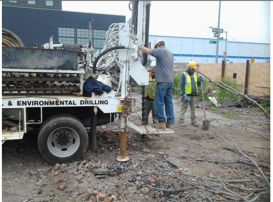
**Photo 4 – C2 Environmental collecting soil borings using a track-mounted Geoprobe™ model 6620DT.**
