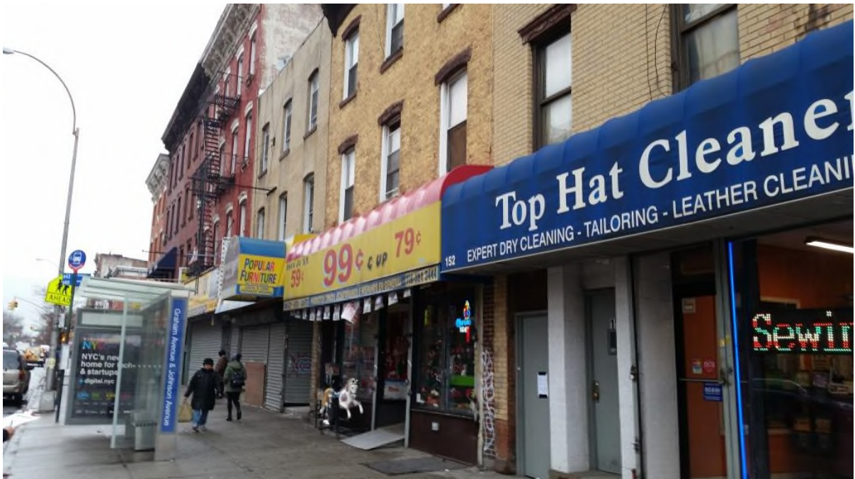
Photograph 2: Near view of the Site and adjoining Top Hat Cleaners operation looking north along the Graham Avenue sidewalk.
