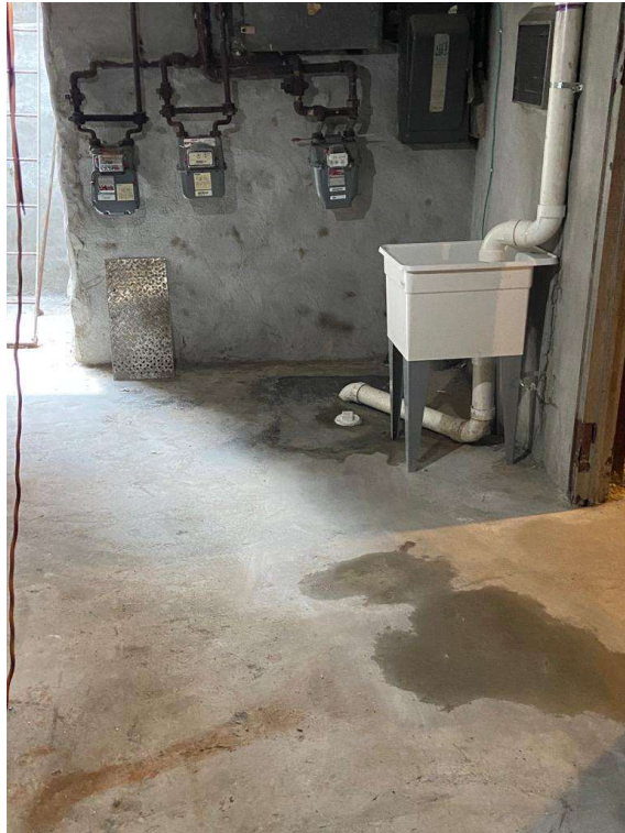
View of new slab and sealed masonry stone walls in partial basement
