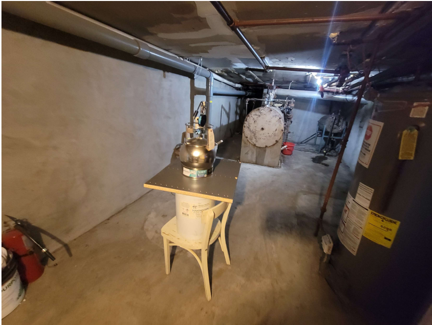
Indoor air sampling in the partial basement
