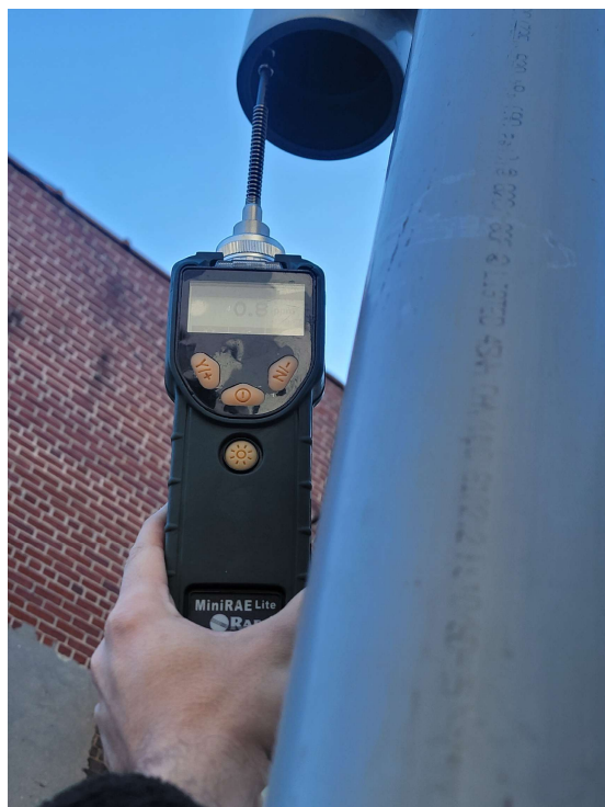
PID reading at SSDS effluent
