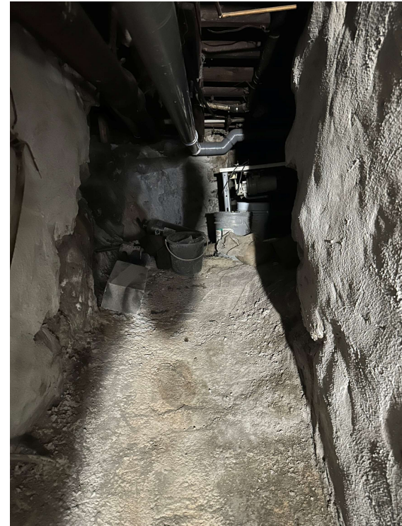
View of new slab and sealed masonry stone walls in crawl space
