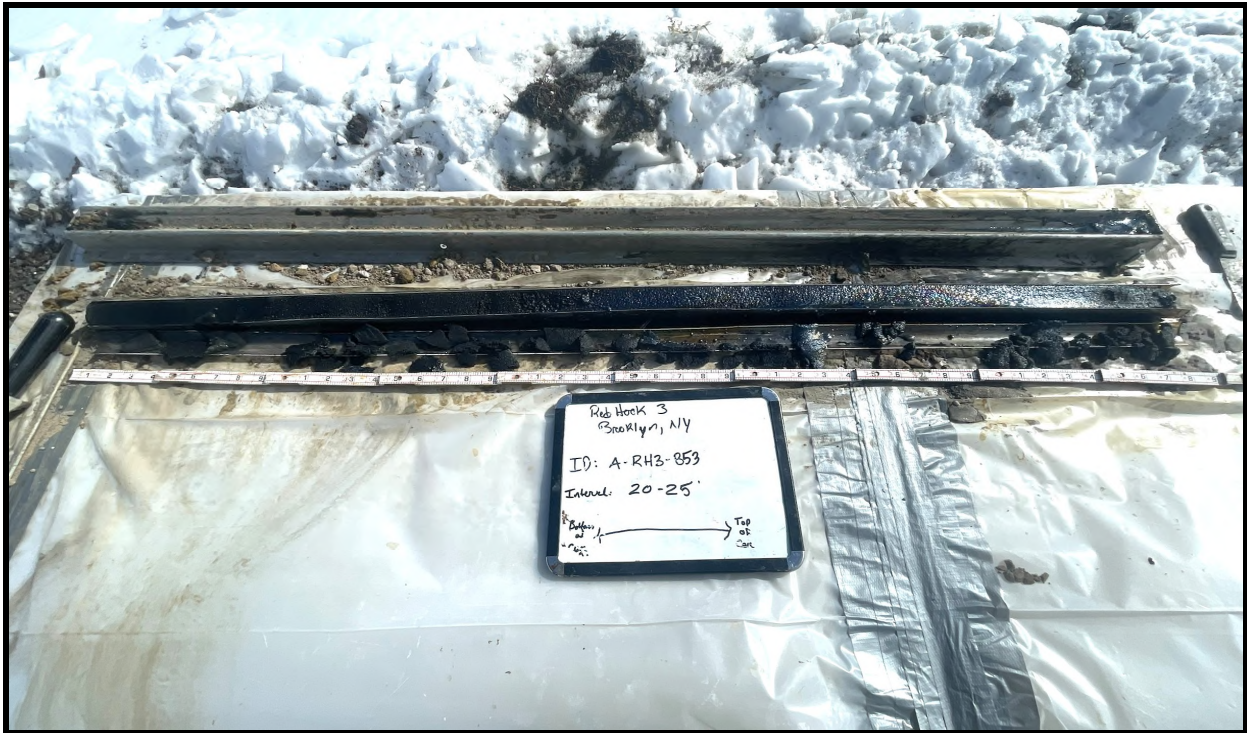
Photo 71: A-RH3-B53 – 20 to 25 feet showing staining
