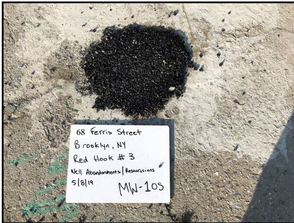
MW-10S Surface Completion with Cold Patch
