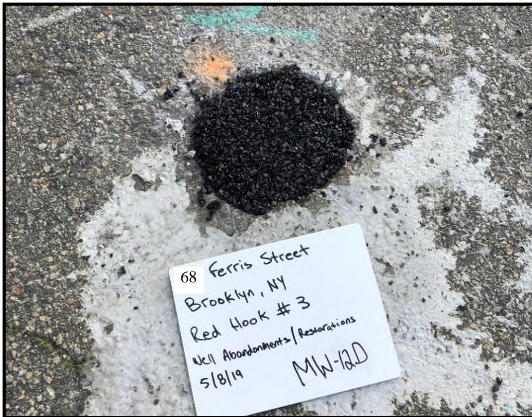
MW-12D Surface Completion with Cold Patch
