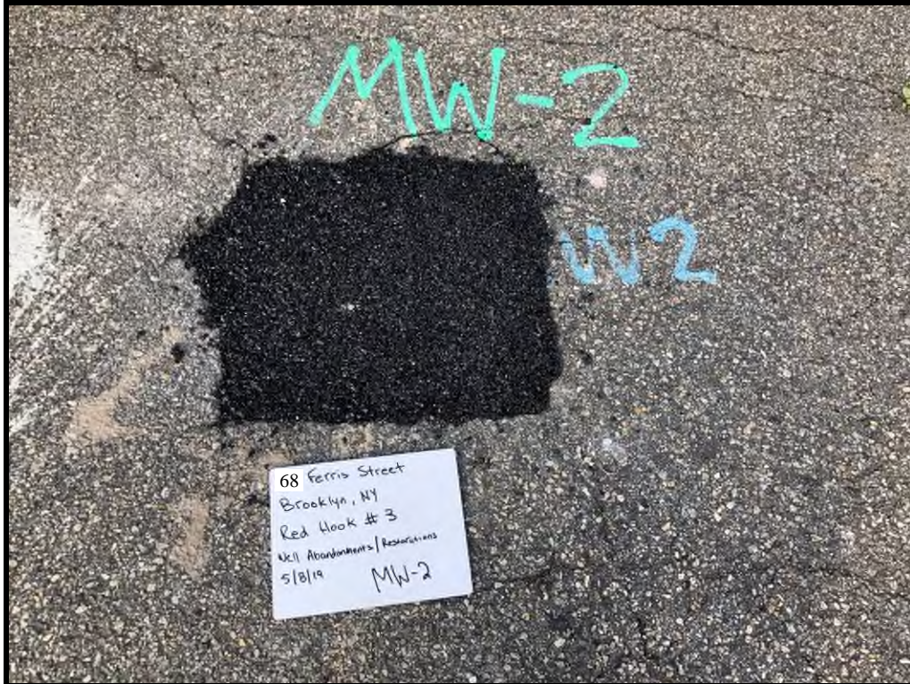
MW-2 Surface Completion with Cold Patch
