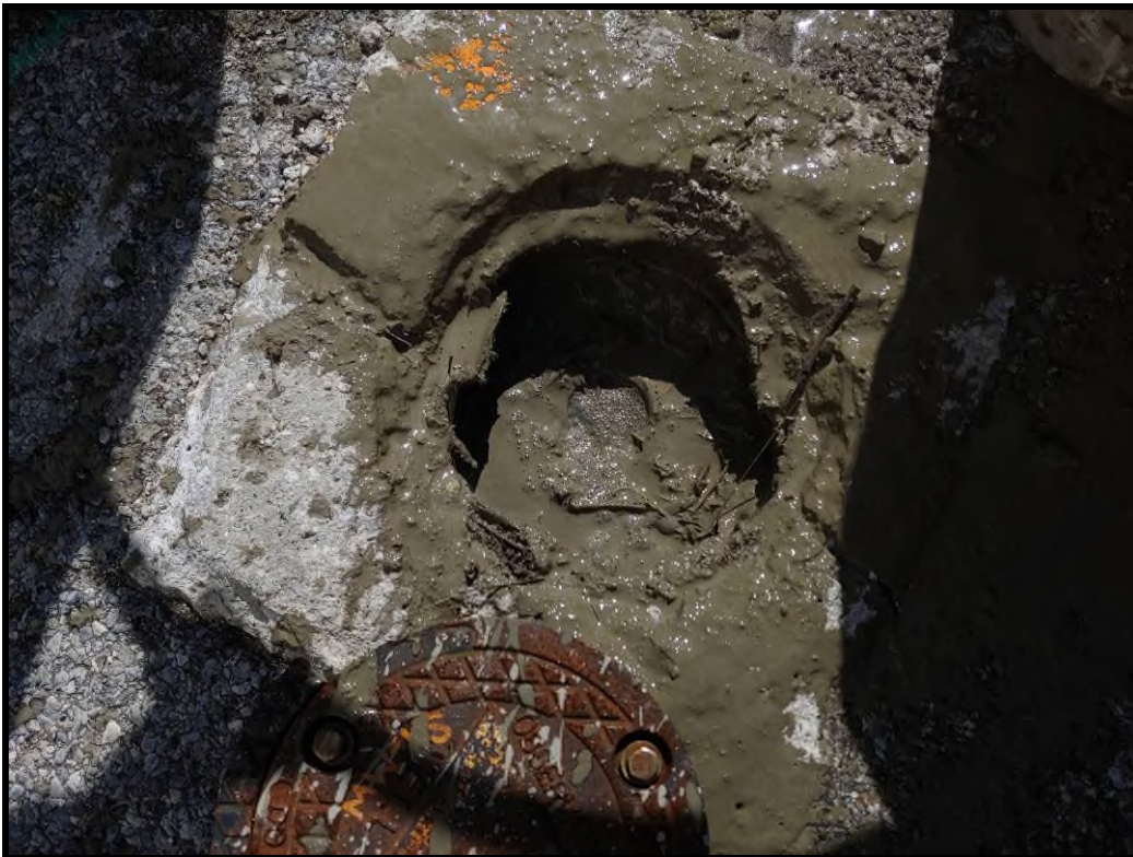
MW-11S with PVC Riser Grouted
