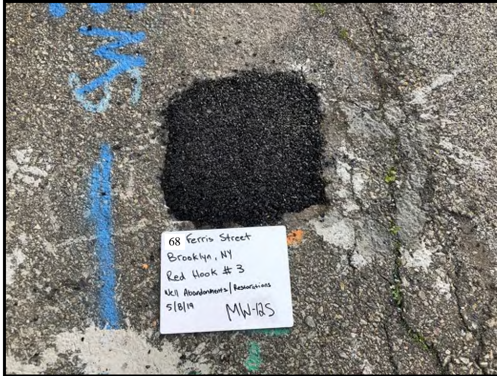
MW-12S Surface Completion with Cold Patch
