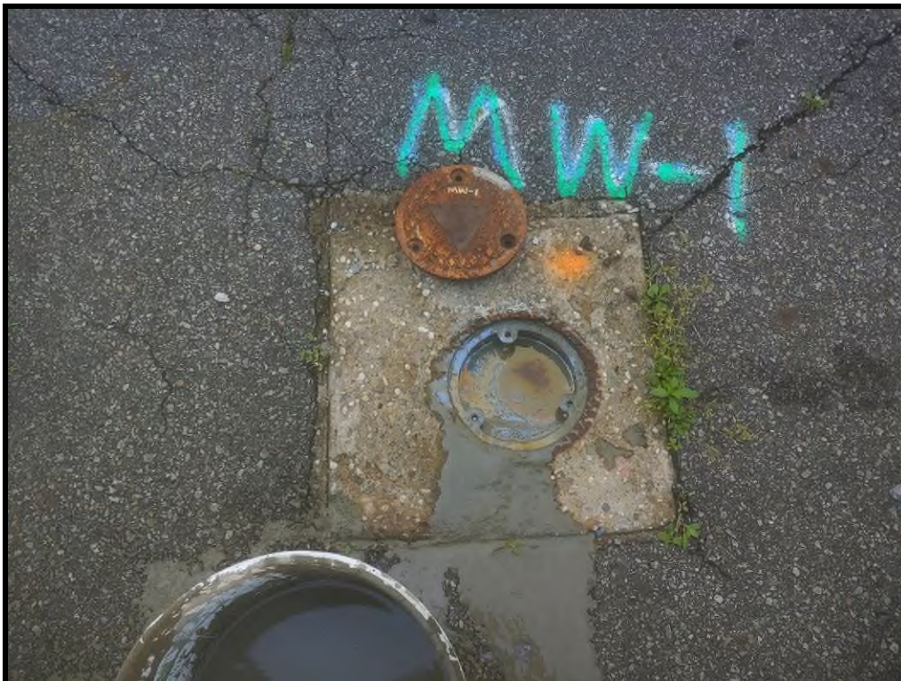
MW-1 with PVC Riser Grouted
