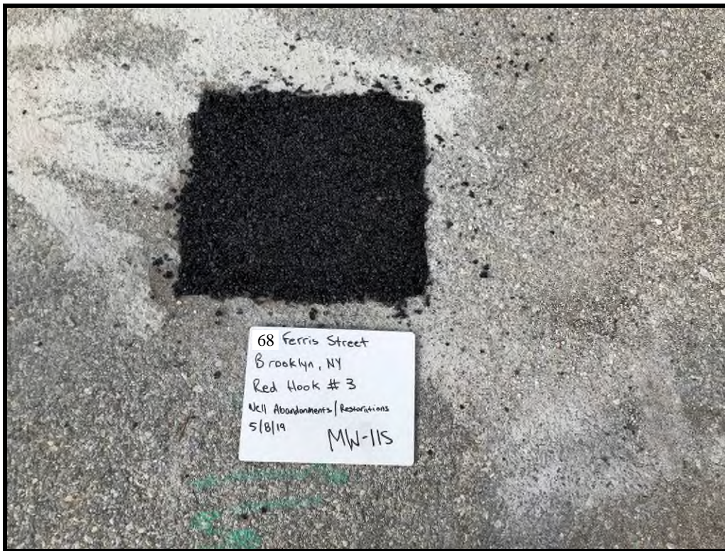
MW-11S Surface Completion with Cold Patch
