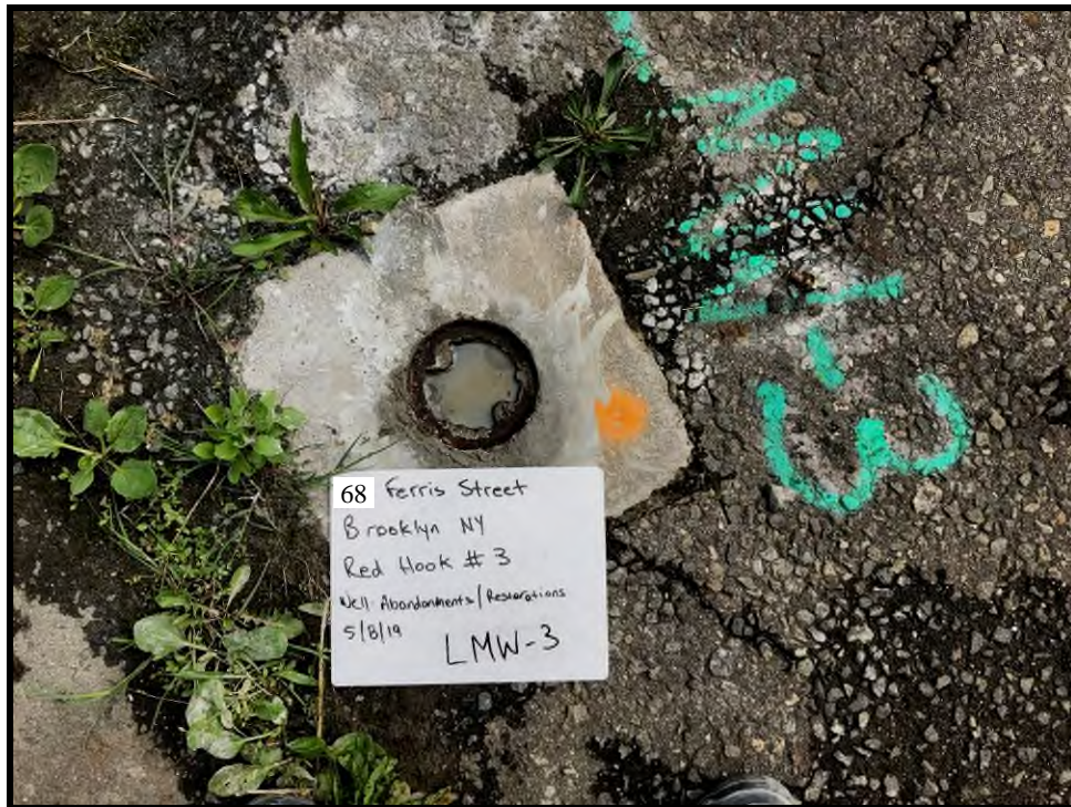
LMW-3 with PVC Riser Grouted
