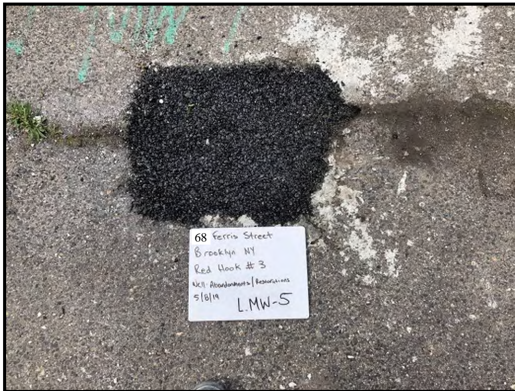
LMW-5 Surface Completion with Cold-Patch
