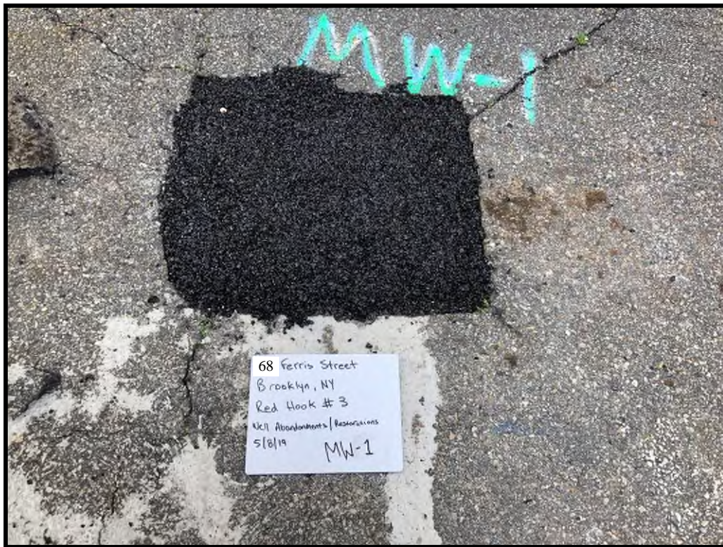
MW-1 Surface Completion with Cold Patch
