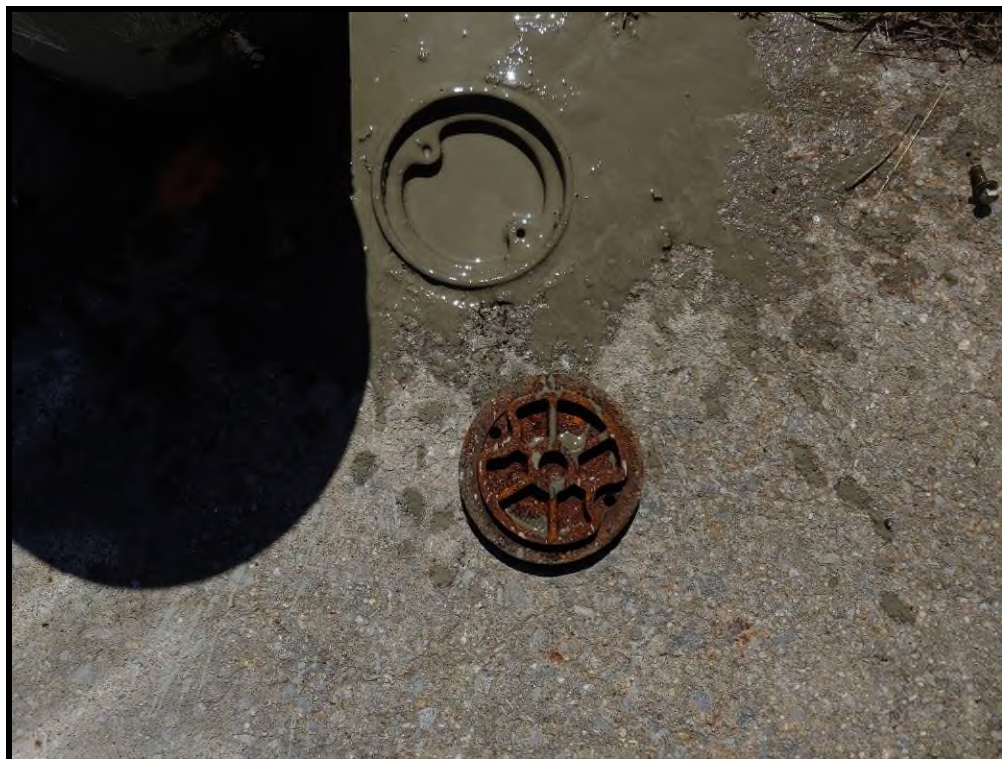
TMW-1 with PVC Riser Grouted
