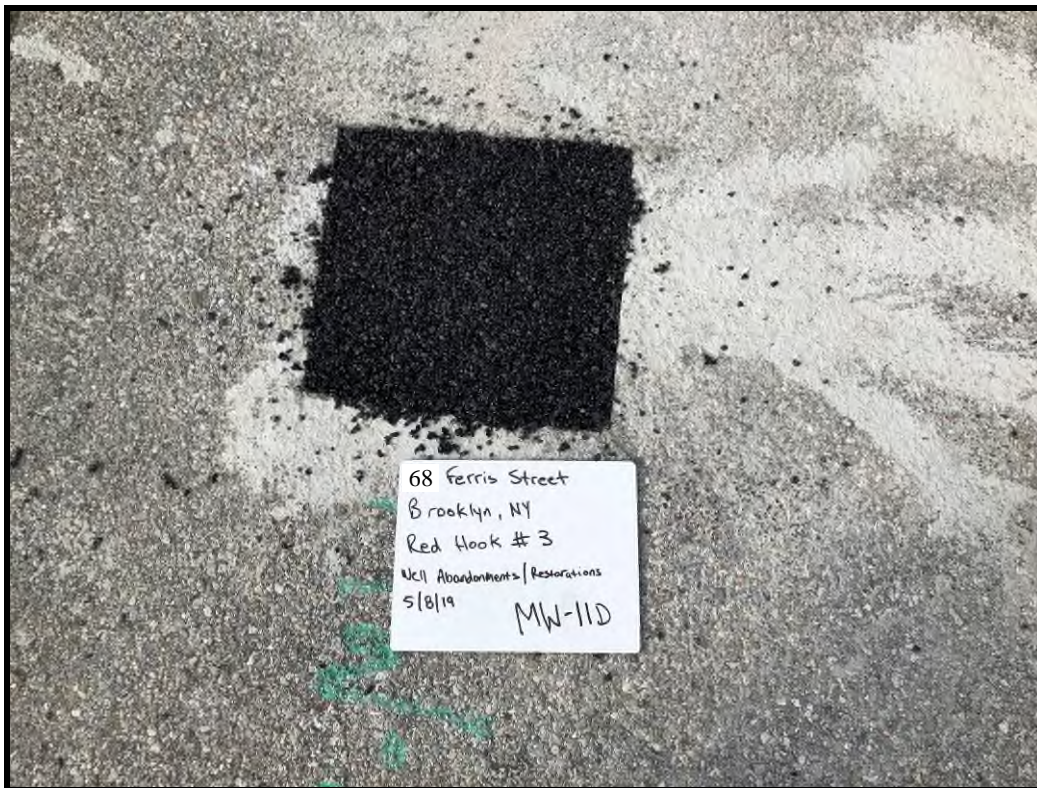
MW-11D Surface Completion with Cold Patch
