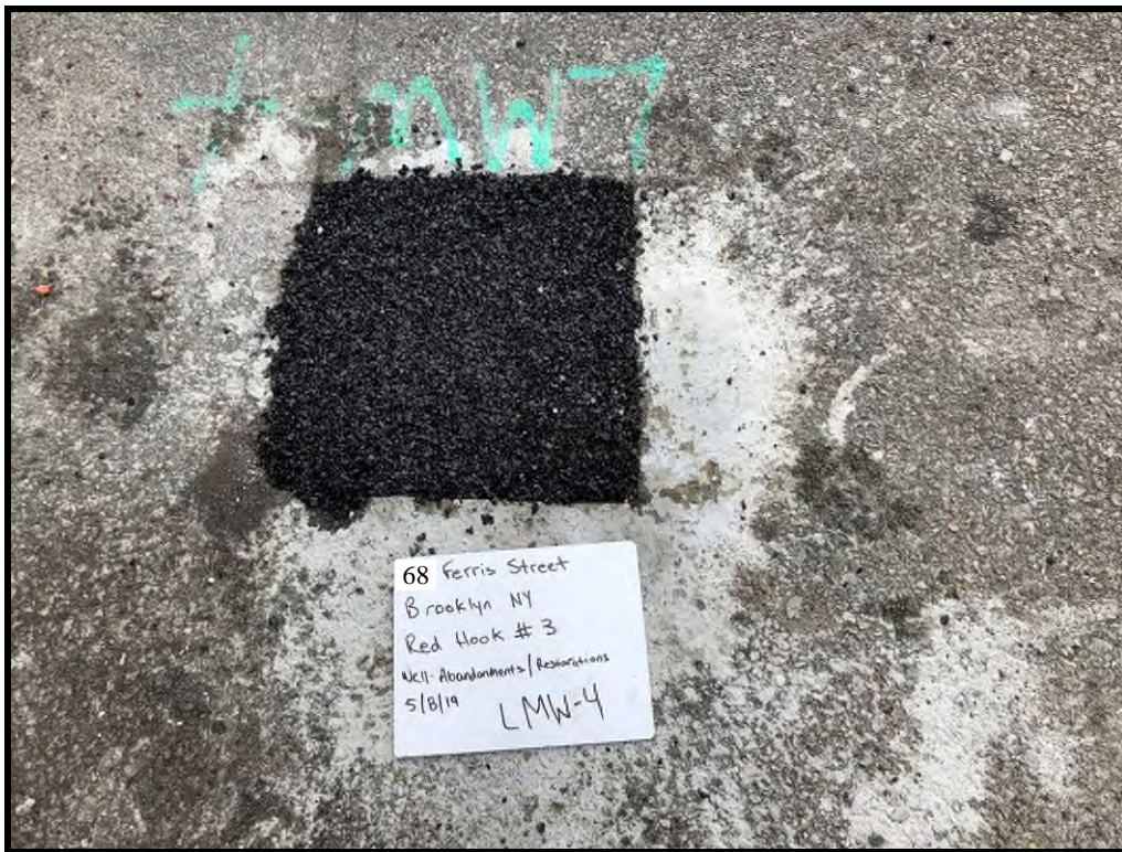
LMW-4 Surface Completion with Cold-Patch
