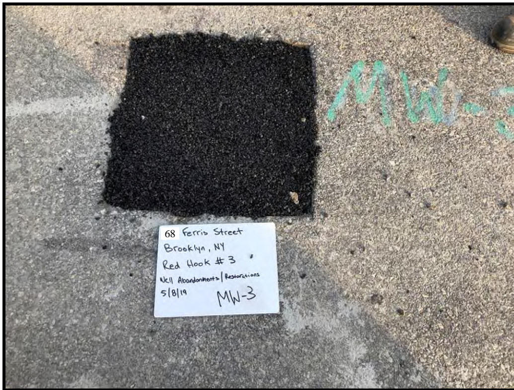
MW-3 Surface Completion with Cold Patch
