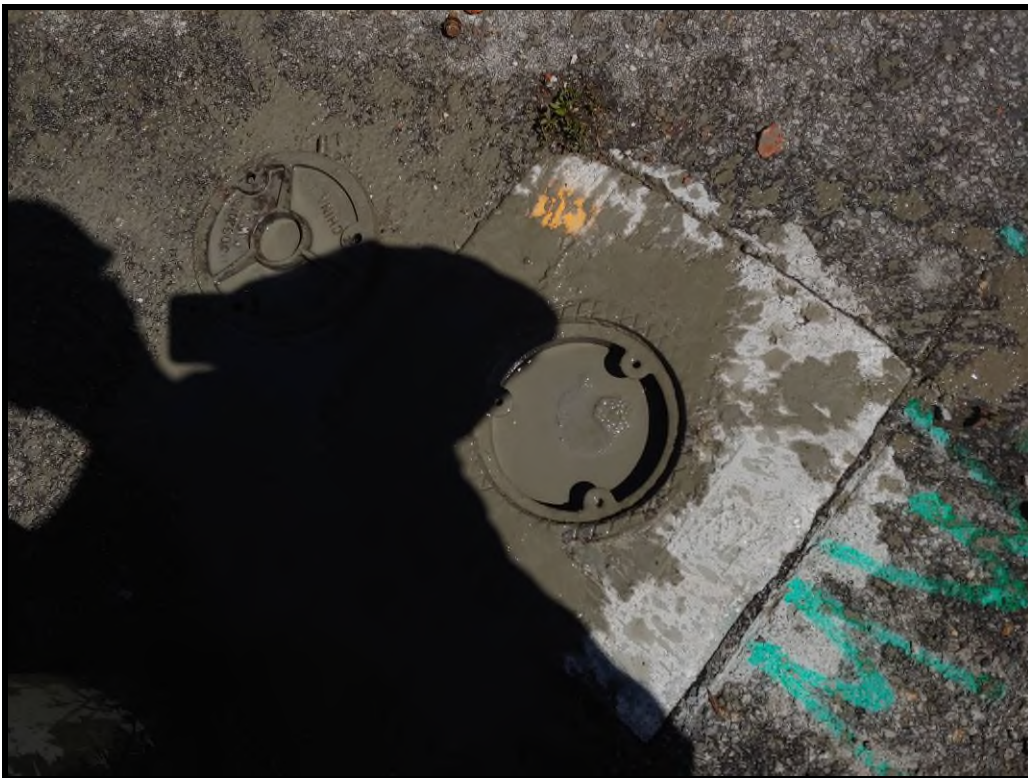
LMW-4 with PVC Riser Grouted
