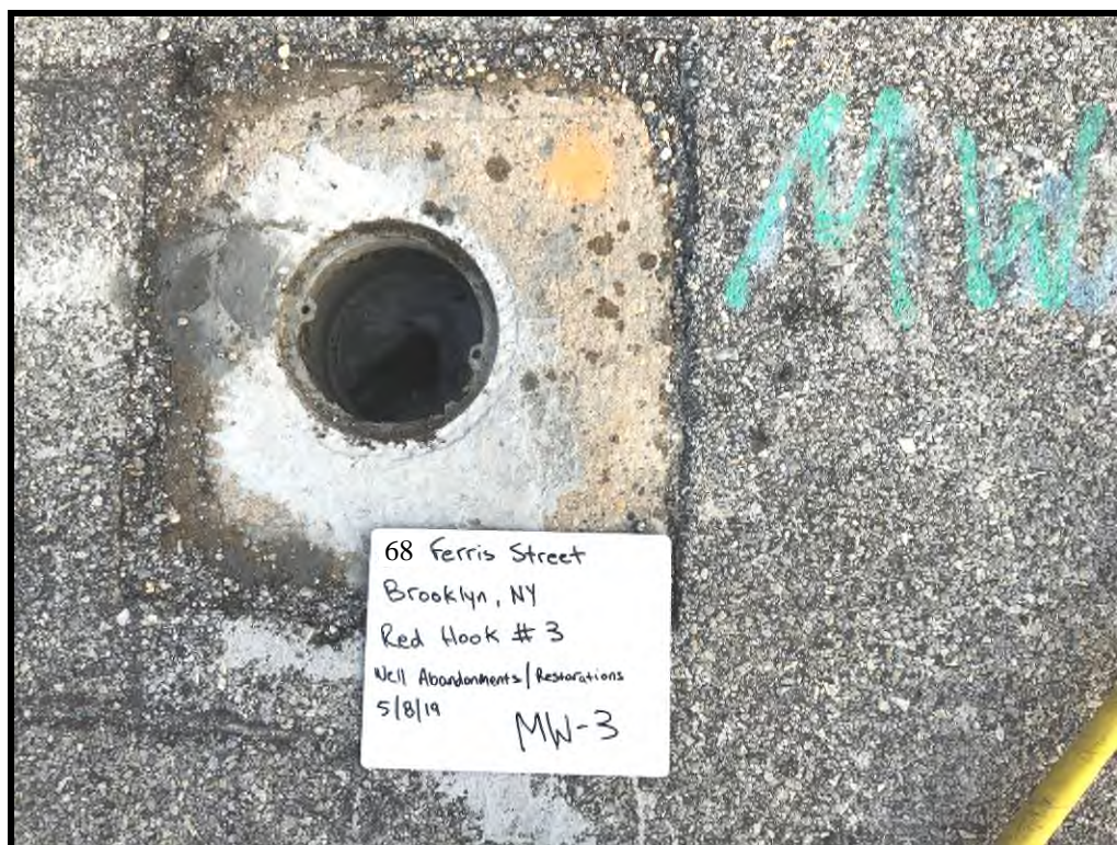
MW-3 with PVC Riser Grouted
