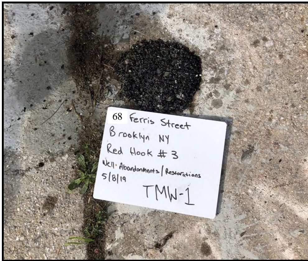
TMW-1 Surface Completion with Cold Patch
