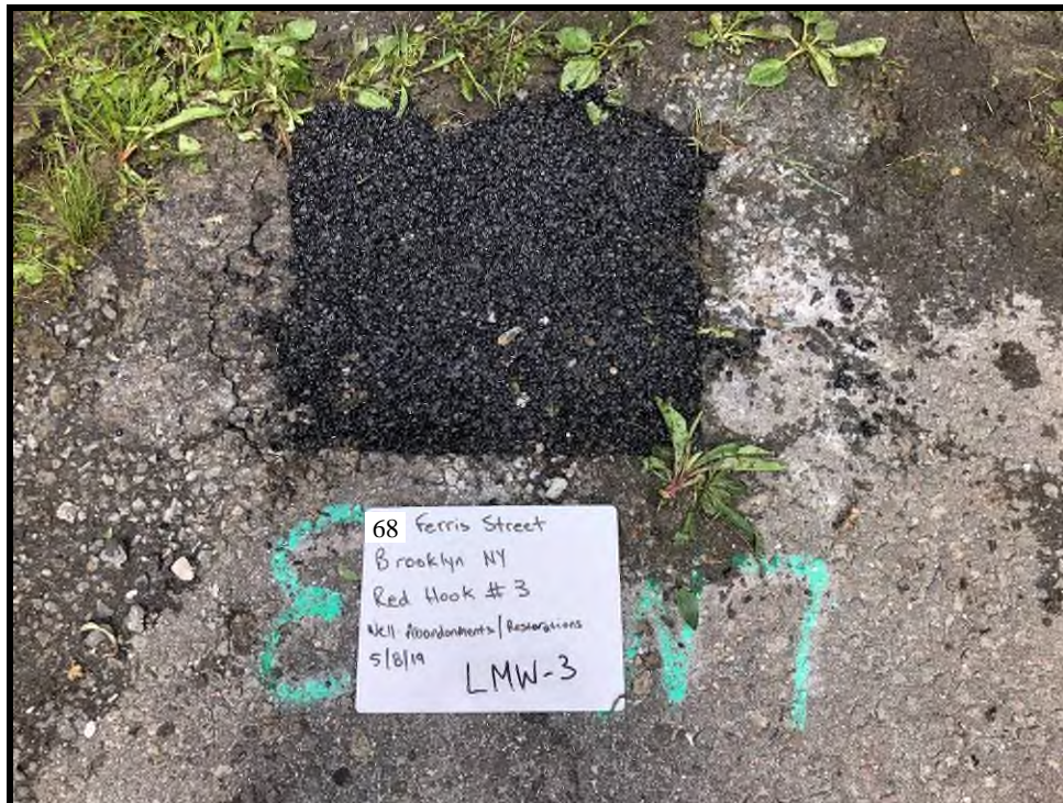
LMW-3 Surface Completion with Cold-Patch
