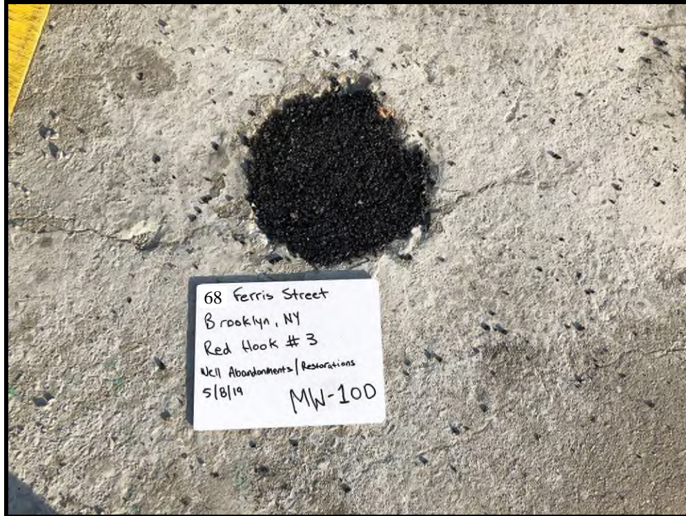
MW-10D Surface Completion with Cold Patch
