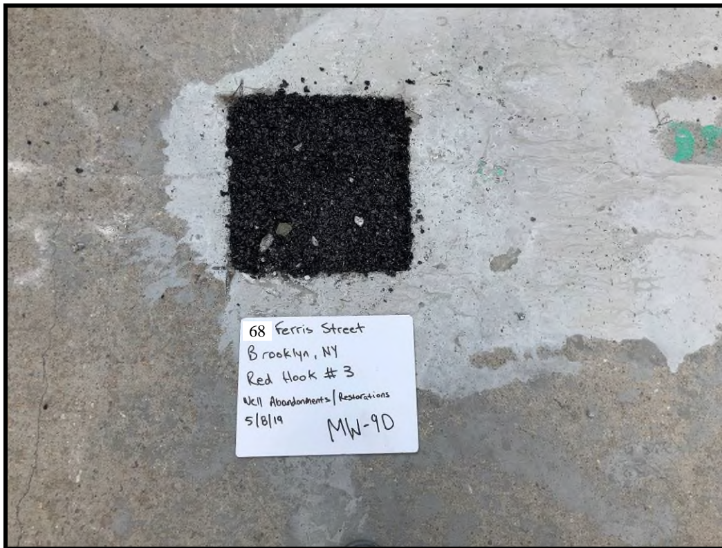
MW-9D Surface Completion with Cold Patch
