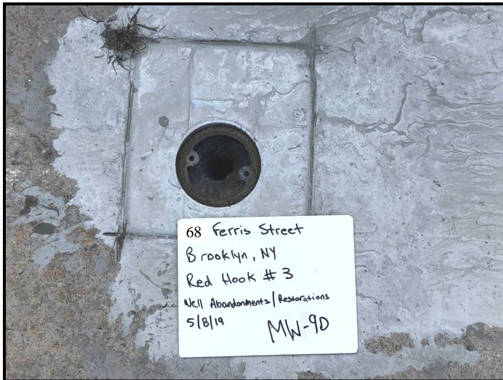
MW-9D with PVC Riser Grouted
