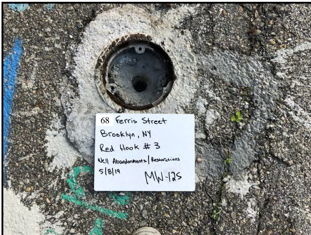
MW-12S with PVC Riser Grouted
