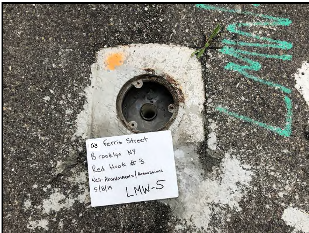
LMW-5 with PVC Riser Grouted
