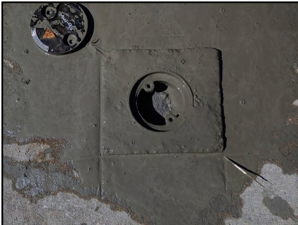
MW-9S with PVC Riser Grouted
