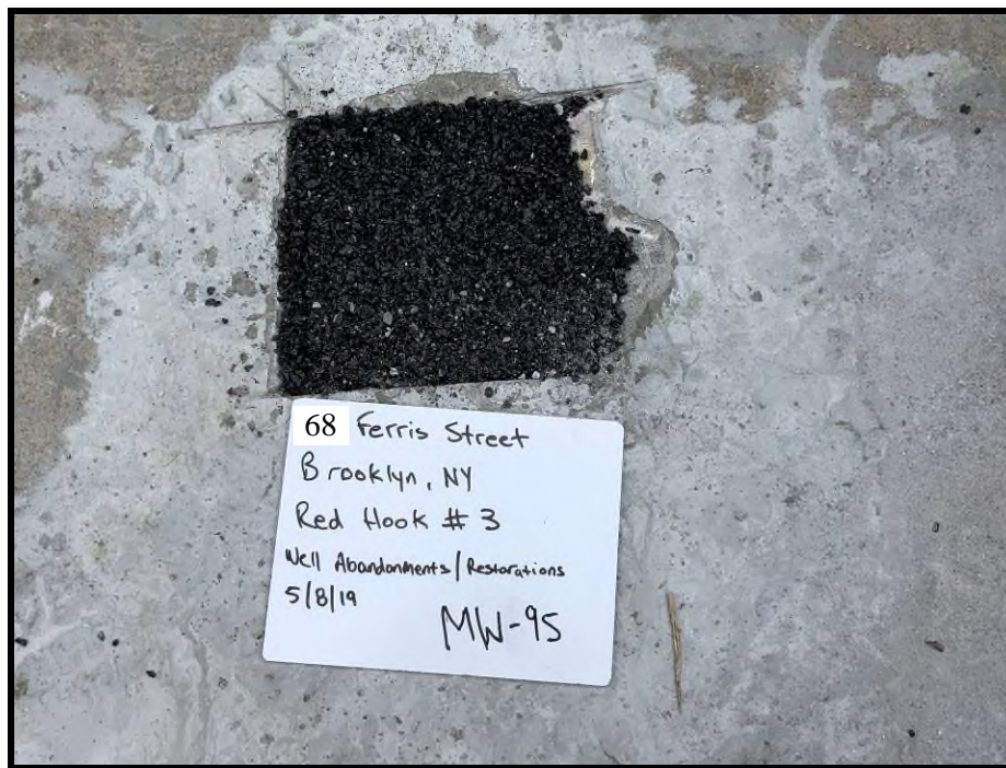
MW-9S Surface Completion with Cold Patch
