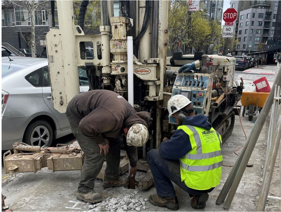
Photograph 7: Eastern Environmental installing monitoring well MW02 (facing east).
