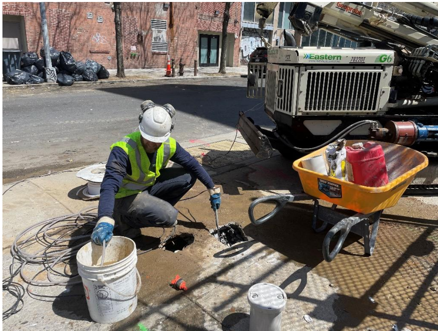
Photograph 8: Developing monitoring well MW01A.
