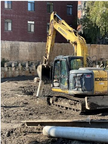
*Photo 3: Excavation and installing new suction point in the middle of the site.*
