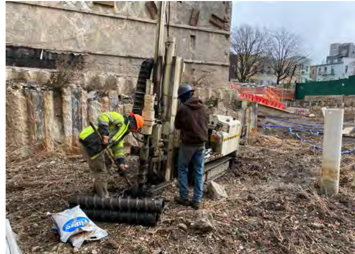
Photo 2: Installation of MW03.
