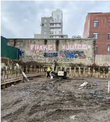
Photo 1: Installation of SB02.
