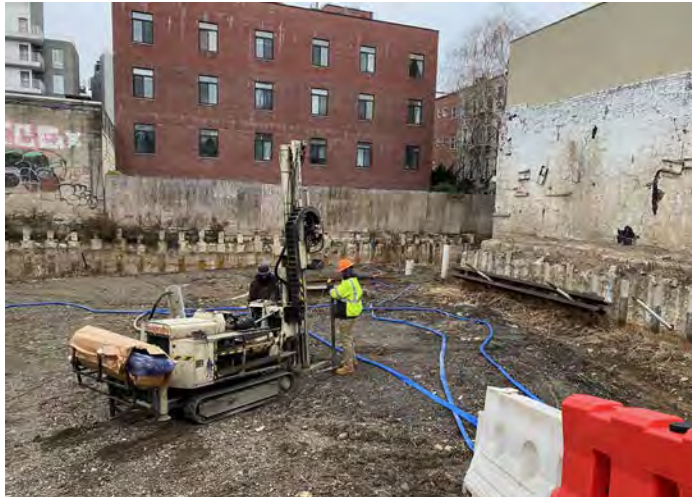
Photo 1: Installation of SB06.
