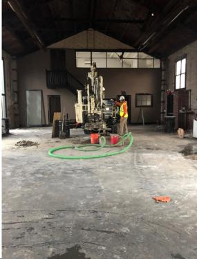
Photo 2: View of the downwind CAMP station during installation of MR-11. Additional absorbent boom was placed by the door to prevent potential off-site migration of fluids.
