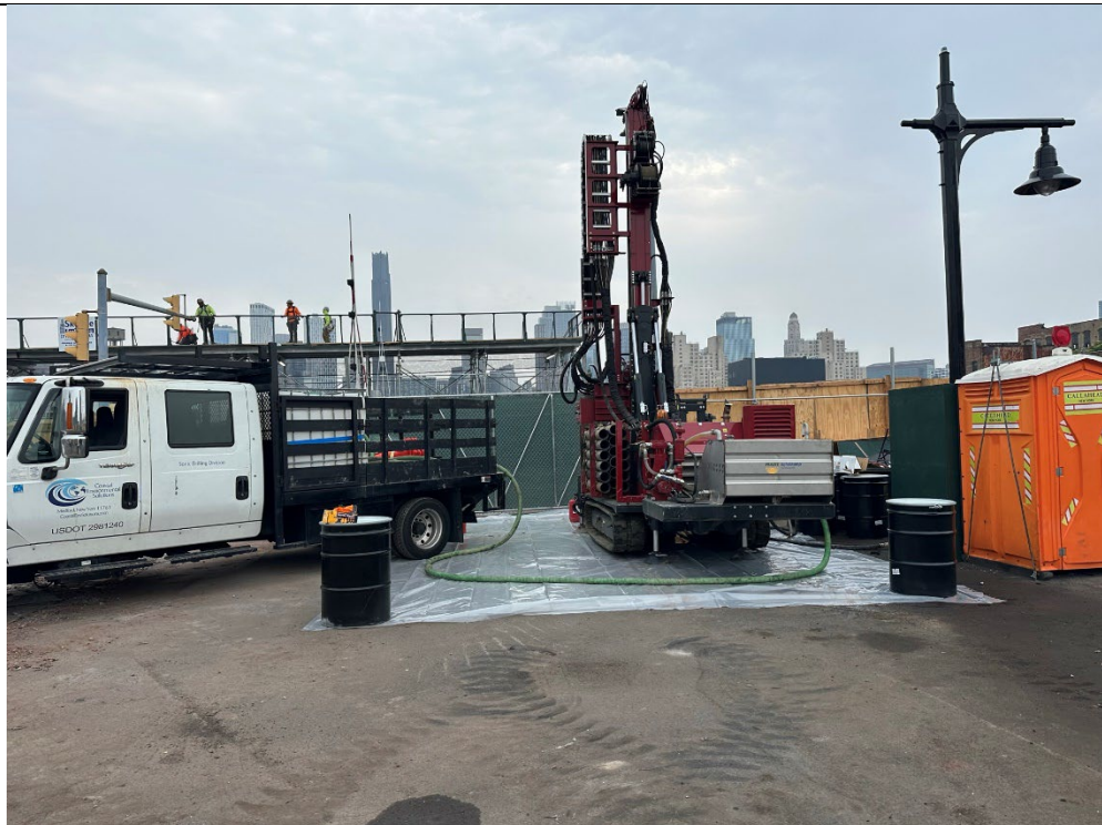
Photo 1: View of Coastal Environmental Solutions mobilizing sonic drill rig prior to drilling DB-1 facing northeast.
